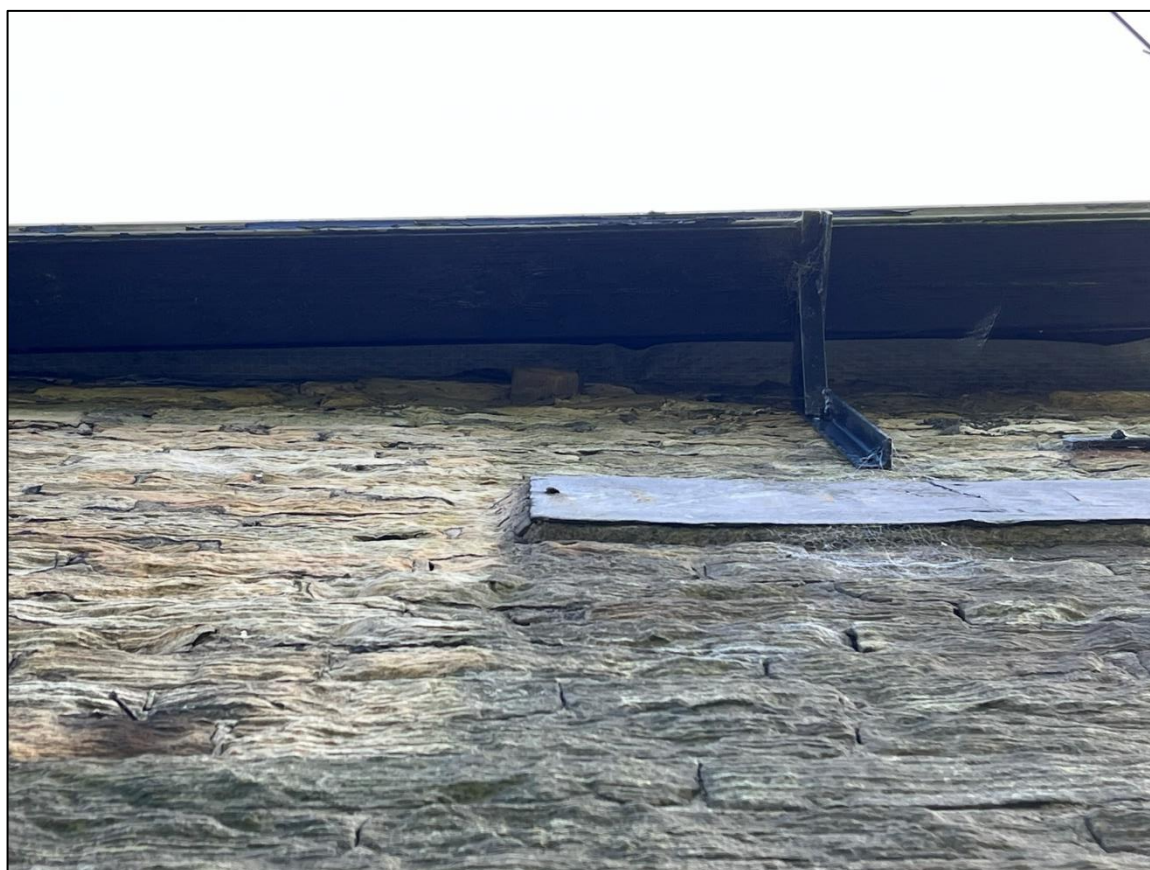
Plate 14 – Open eaves located on Sections B and C
