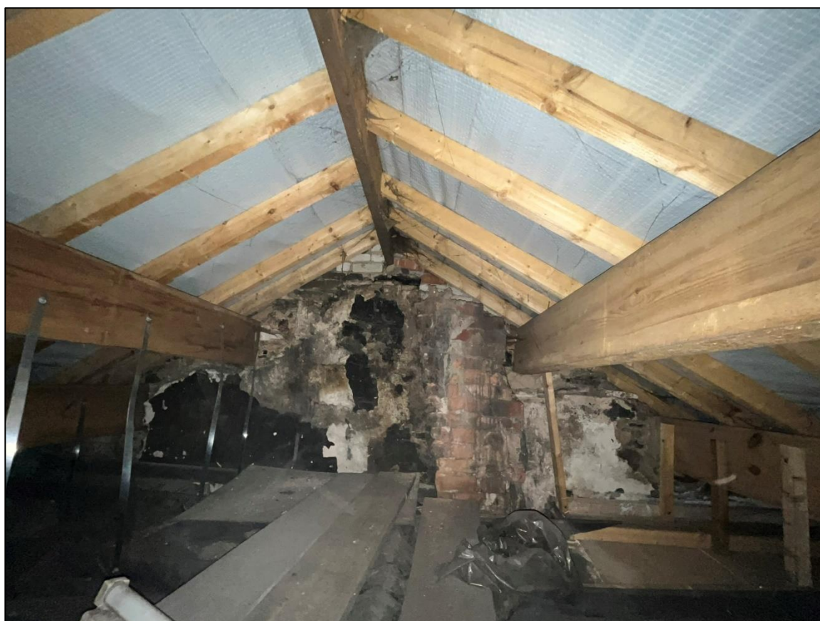
Plate 8 – Character of the loft spaces above Section B
