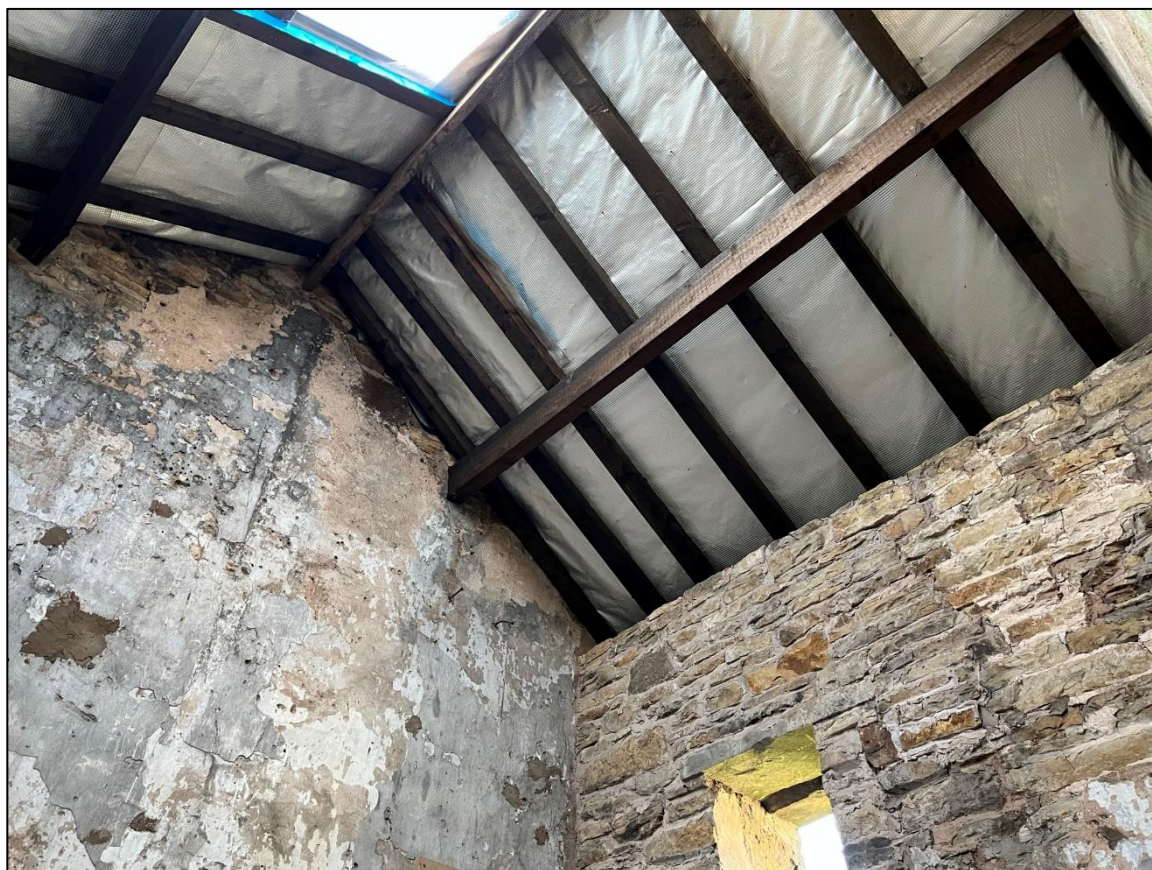
Plate 9 – Internal character of the loft space of Section C
