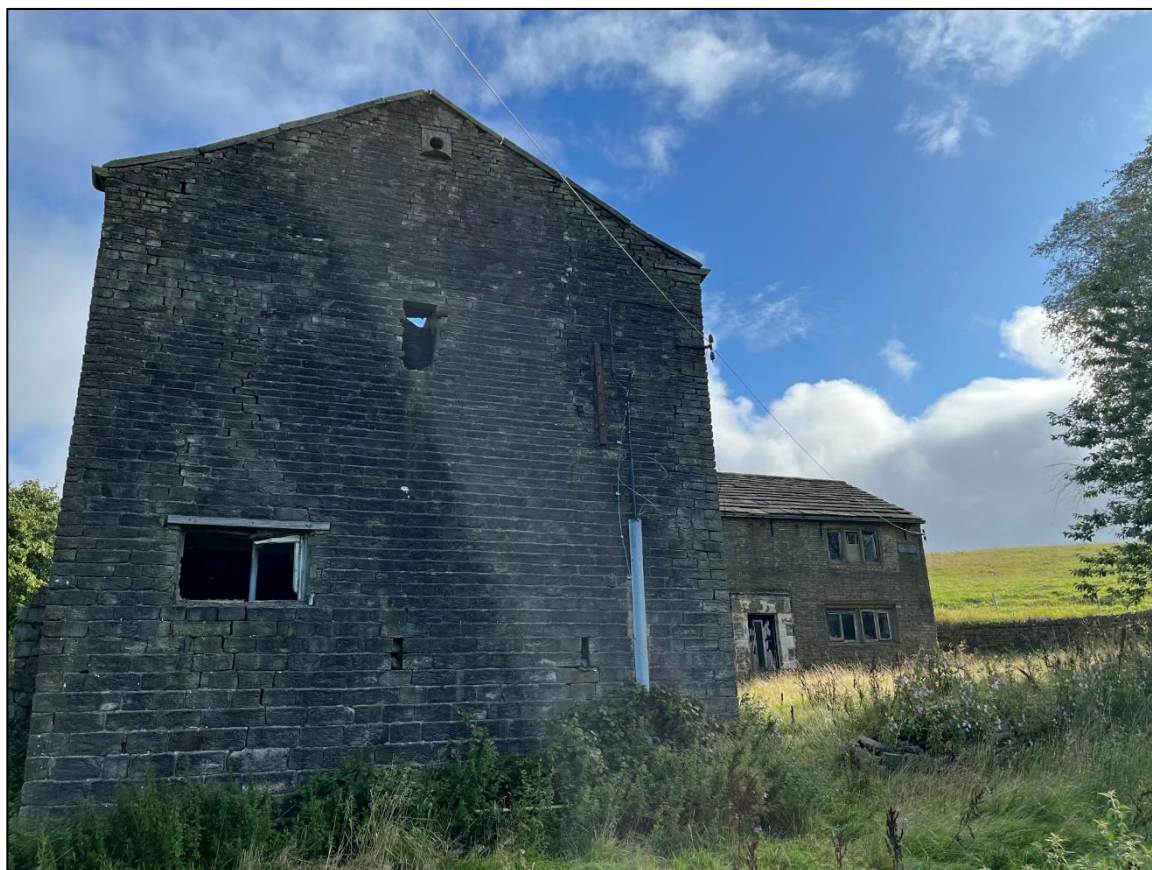
Plate 5 – South-western aspect of the structure, with Section D to left and Section B to right
