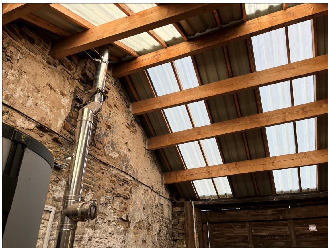
Plate 6 – Internal character of Section A
