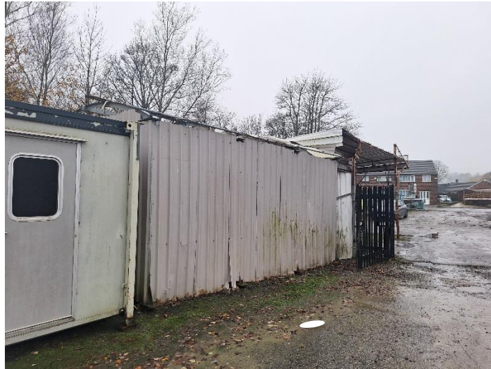
PLATE 21 SHOWING NORTH-EAST ASPECT OF S2
