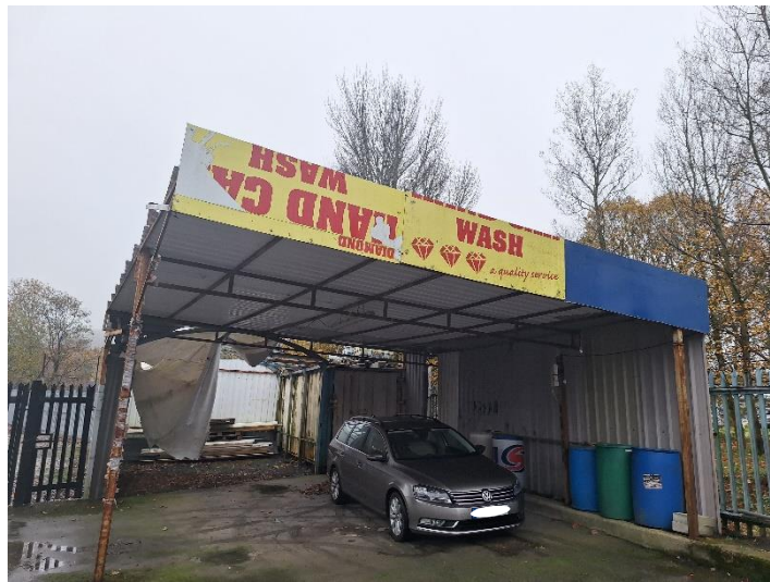
PLATE 19 SHOWING NORTH WEST ASPECT OF S2
