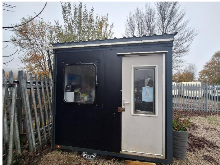
PLATE 16 SHOWING NORTH-EAST ASPECT OF B4
