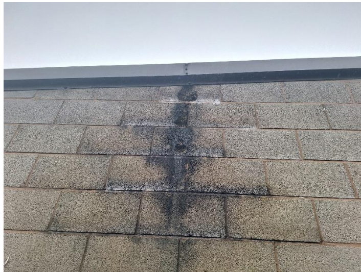
PLATE 6 SHOWING DAMAGED BRICKWORK ON NORTH-EAST ASPECT
