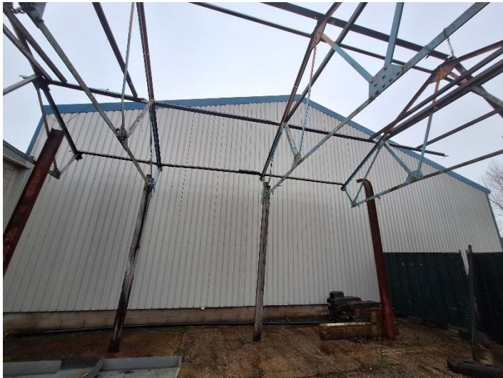
PLATE 12 SHOWING SOUTHERN ASPECT OF B2
