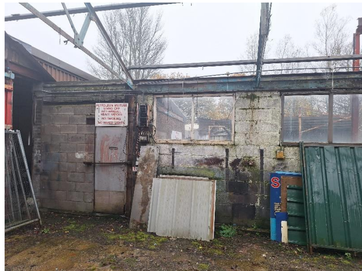
PLATE 18 SHOWING NORTH-EAST ASPECT OF S1
