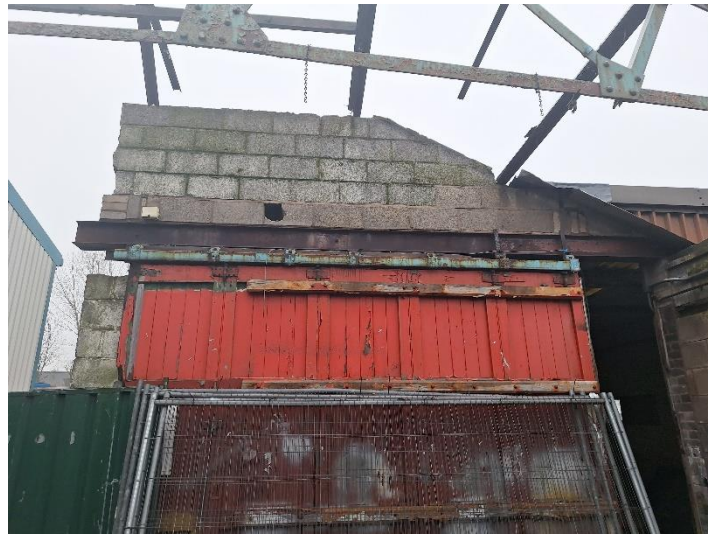
PLATE 1 SHOWING NORTH-WEST ASPECT OF B1
