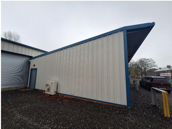
PLATE 14 SHOWING NORTH-EAST ASPECT OF B3
