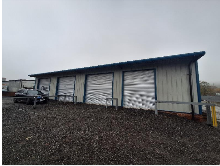
PLATE 13 SHOWING NORTH-WEST ASPECT OF B3
