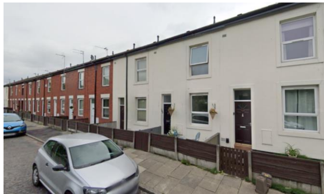
Terrace Housing Bamford Road
