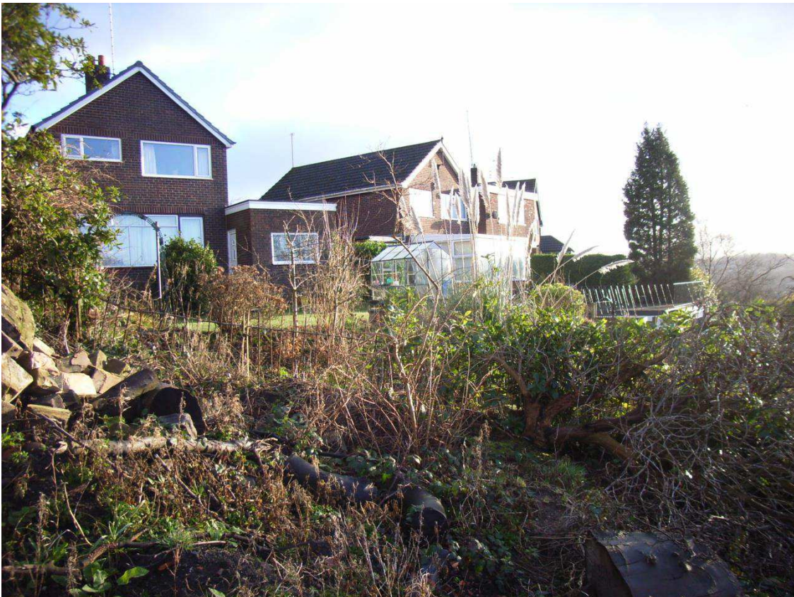
Fig. 2 – Rear elevation, Links View
