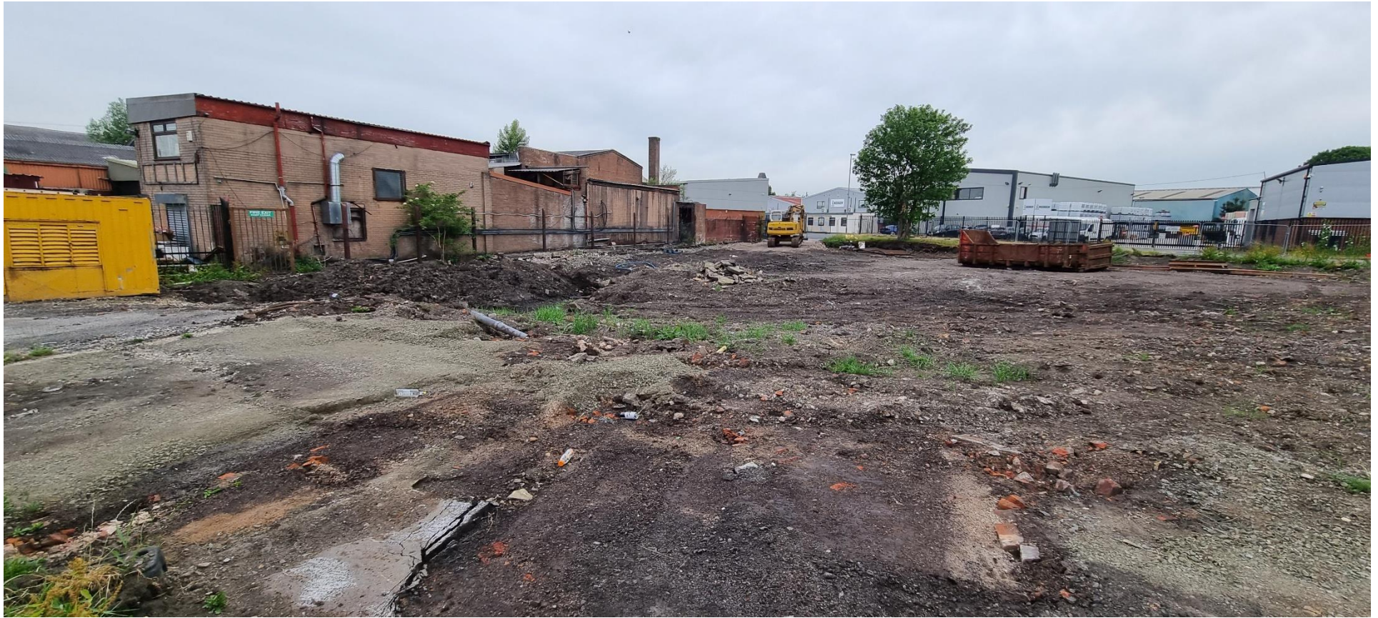
Figure 4: View of the site from Crawford St. boundary displaying the adjoining properties, the existing tree to north and industrial units along Dodgson Street
