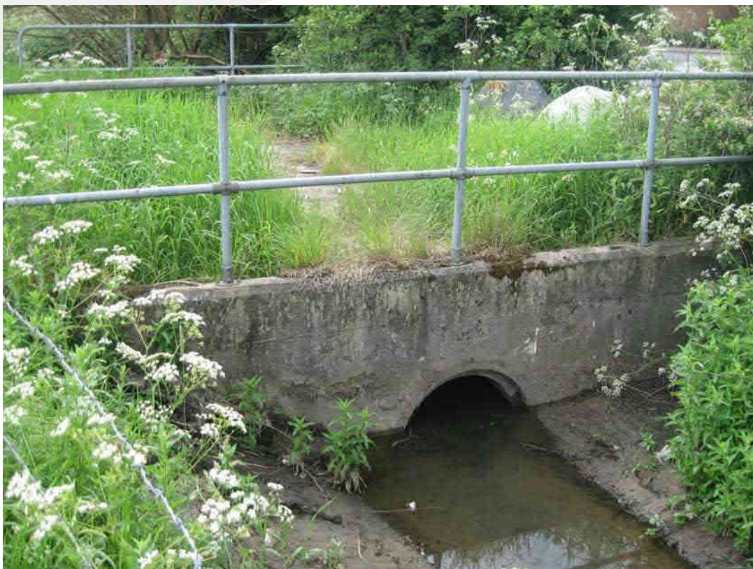
Figure 16: Hydraulic Structure crossing Existing Ditch
