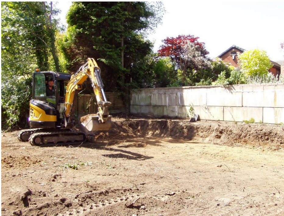
Two views of site clearance area with ground taken down to formation level for detached garage to plot 2.
