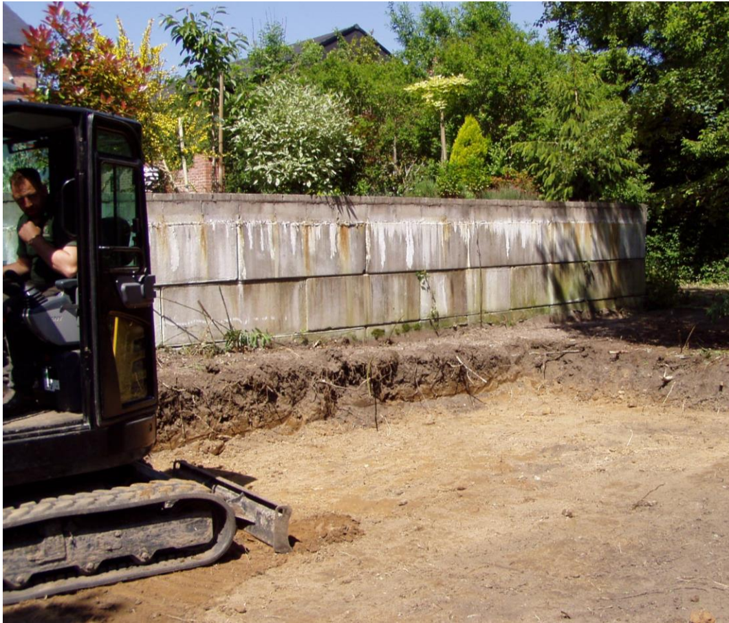
Close up view of levelled area in location of detached garage to plot 2.
