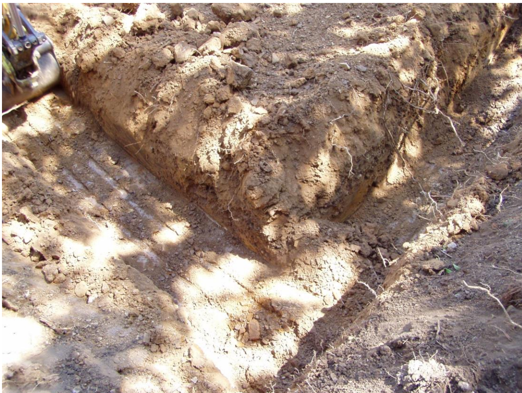
Two views of foundation trench excavation showing very stiff clay over weathered bedrock (very stiff to hard shale) as noted in site investigation report.
