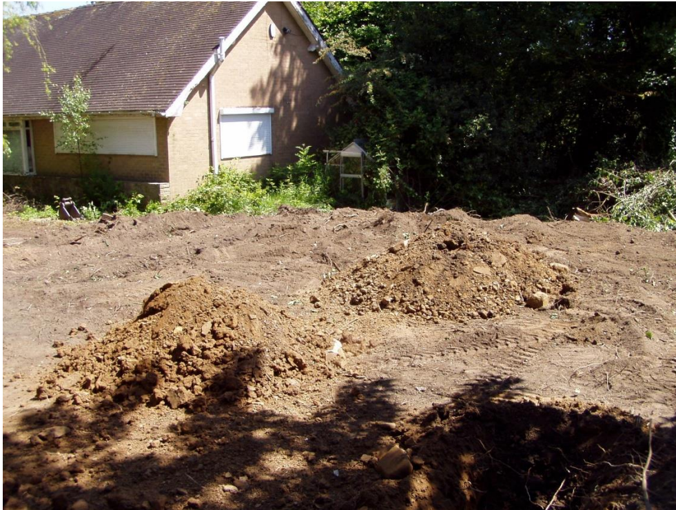
View towards existing bungalow – used as temporary site facilities – showing piles of excavated material.
