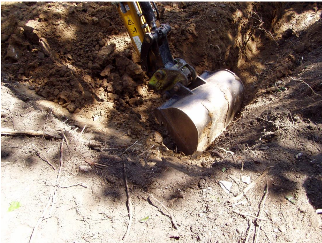
Excavator 'breaking ground'
