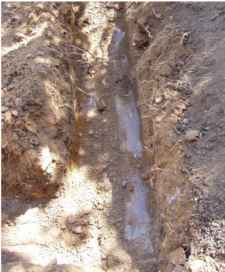
Bottom of foundation trench.
