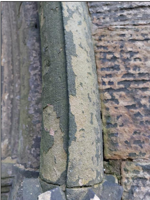
Fig.4 – Contour scaling to stone around tower door opening. De-frass.
