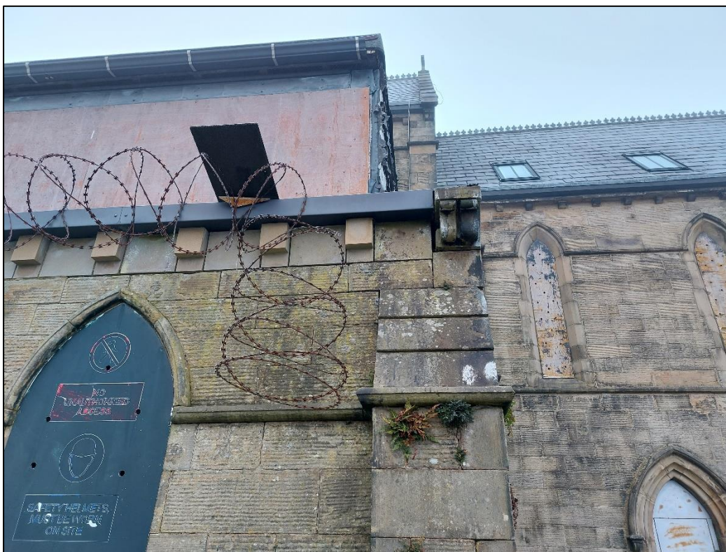
Fig.12 – Algal growth to be removed.
