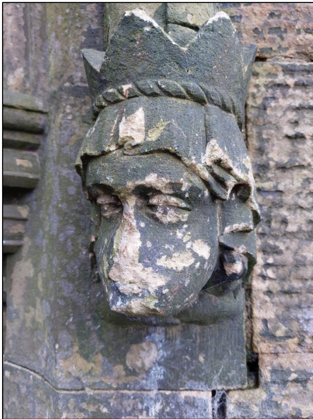
Fig.2 – Carving present to right hand side tower door. To be used as an historical reference for the reinstatement to the left-hand side
