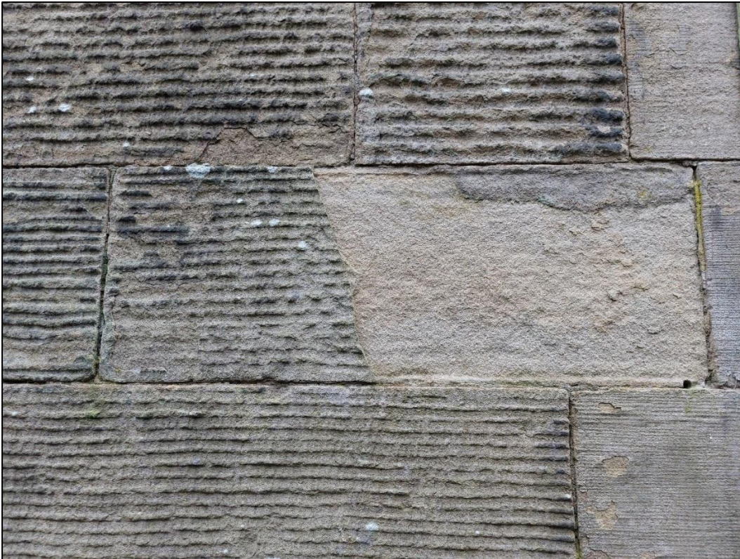
Fig.25 – Contour scaling on isolated block to west elevation. De-frass and remove loose stone.
