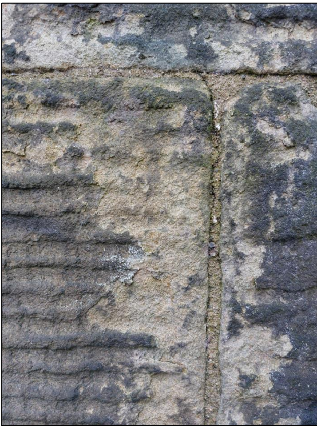
Fig.8 – Contour scaling to stone generally. No work proposed.
