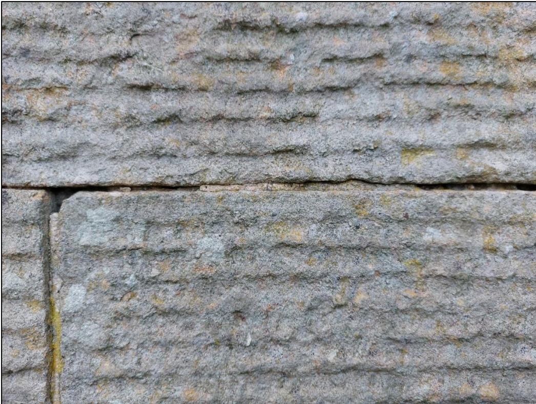
Fig.17 – Photograph to show narrow joints in blocks.
