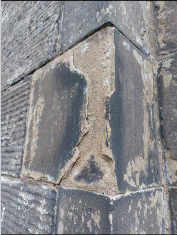
Fig.7 – Contour scaling to quoin block. Proposed to de-frass.
