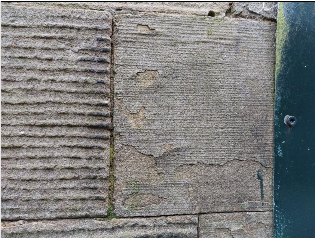
Fig.26 – Contour scaling on isolated quoin block to west elevation. De-frass.
