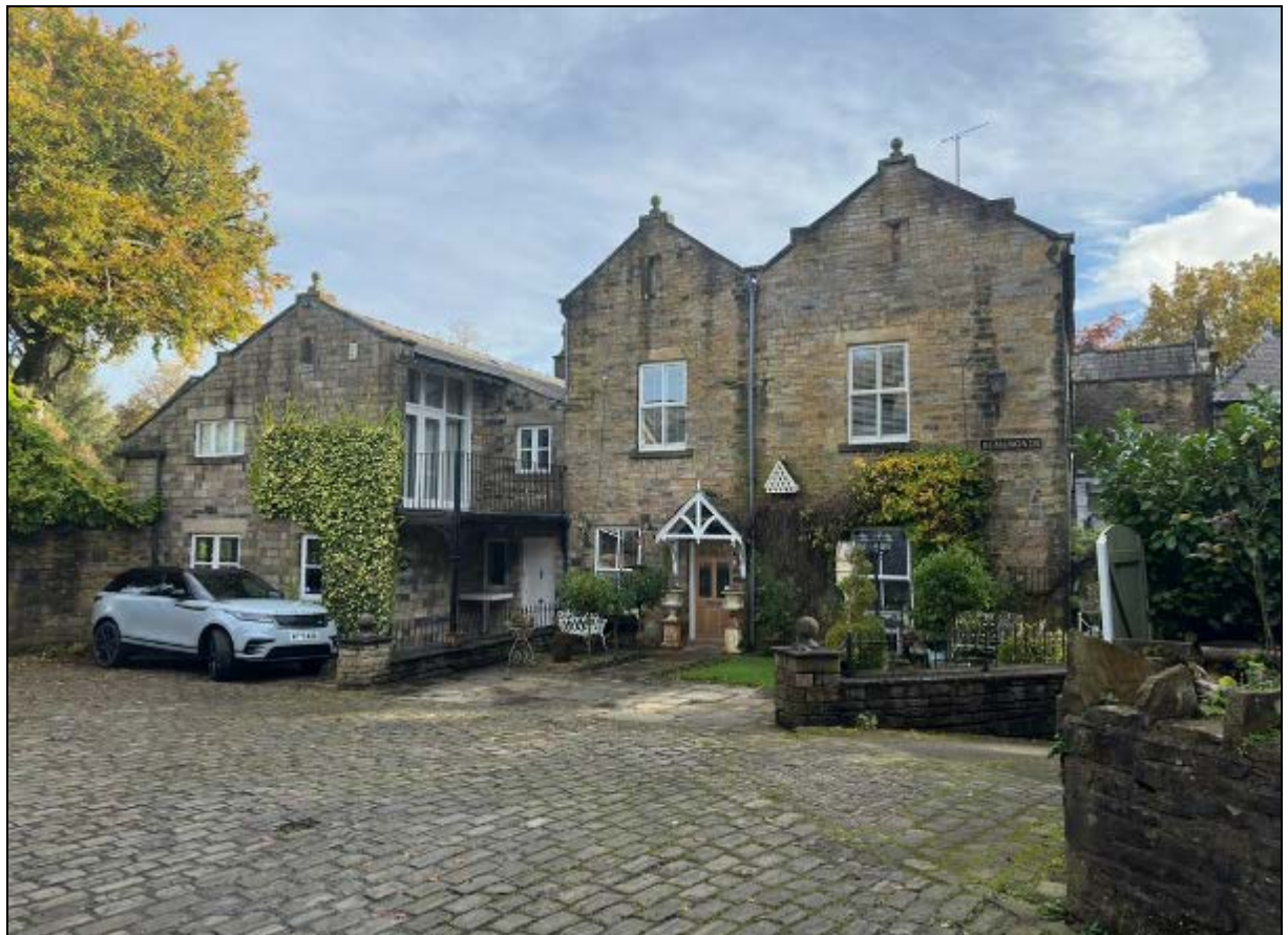
2. View from the courtyard toward number 5, which is within the twin-gabled former kitchen wing of Beaumonts
