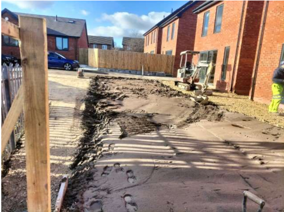
View west from Plot 6 towards Plot 4 across rear garden areas.
