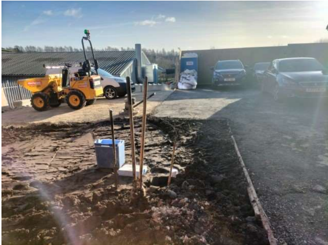
Plot 4 rear garden looking south towards rear car park.
