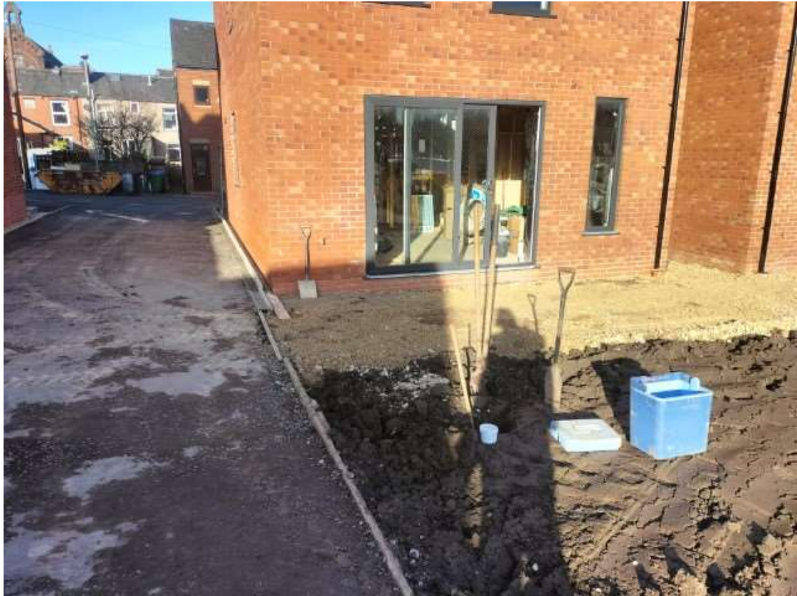
Rear garden of Plot 4, looking towards rear elevation of dwelling. Patio slabs remain to be placed.
