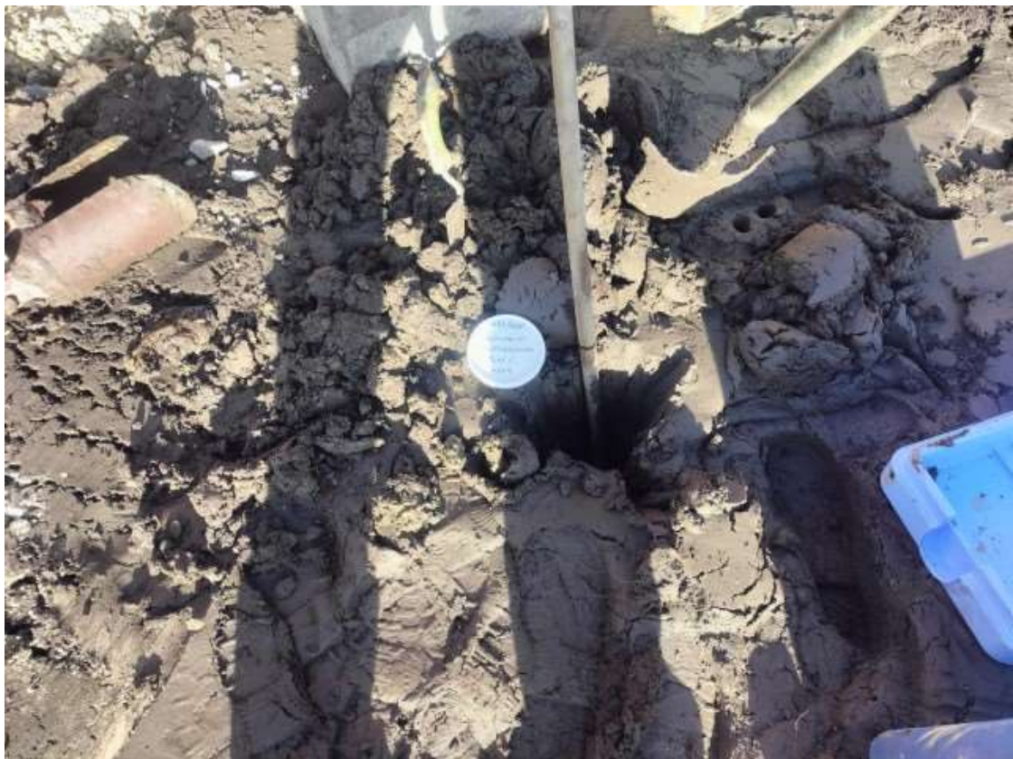
Hand Dug Pit HDP4, Plot 5.
