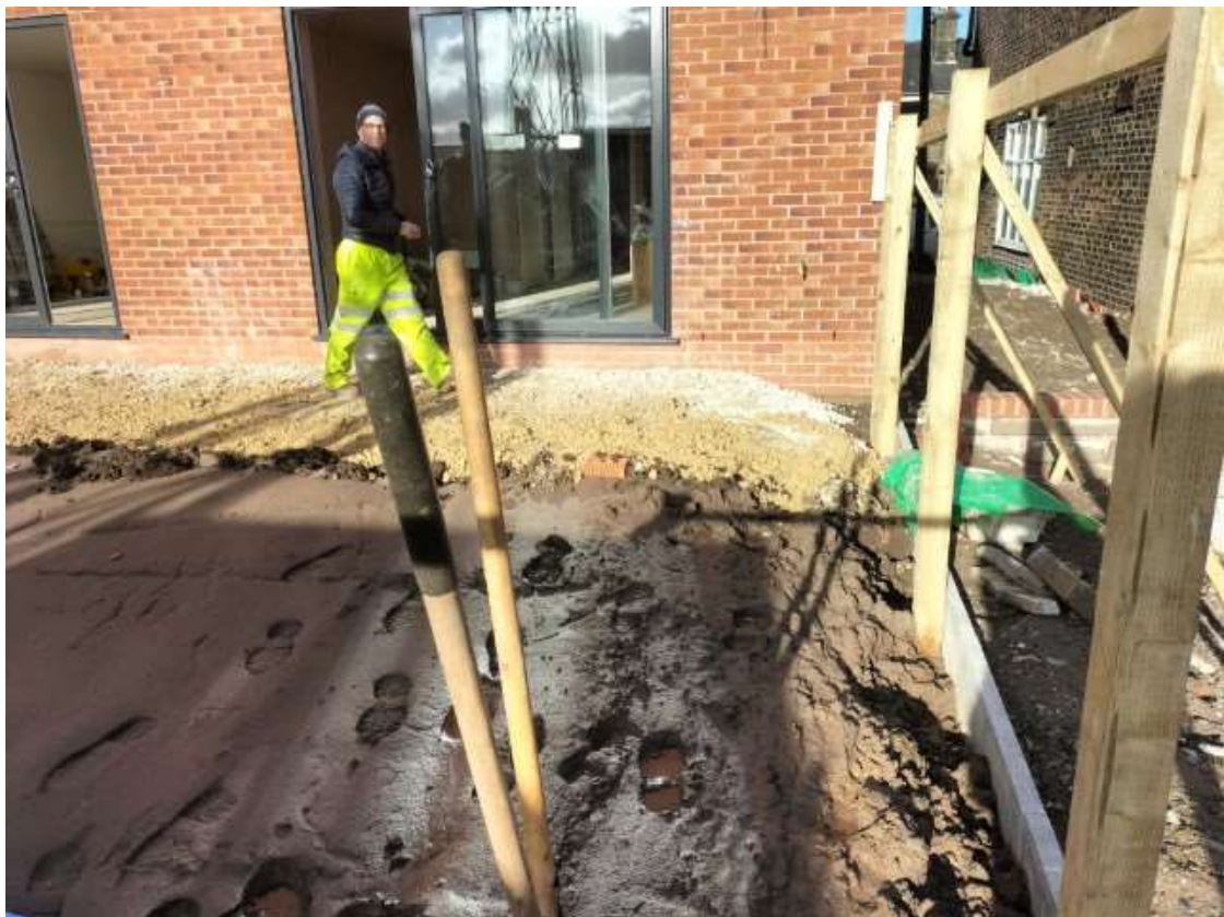
Plot 6 looking north to rear elevation of dwelling.
