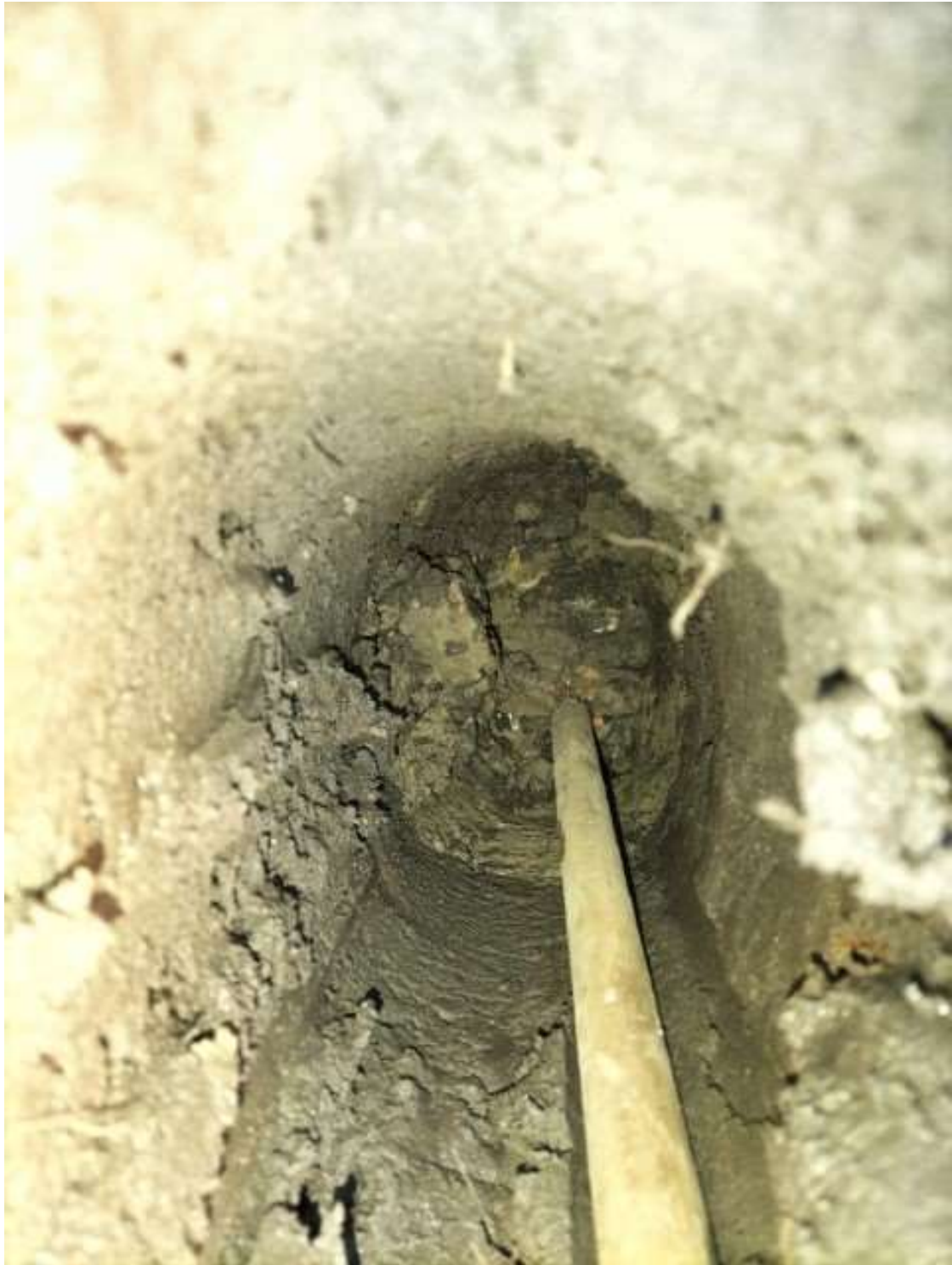
Hand Dug Pit HDP2, Plot 6.
