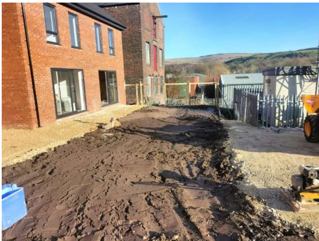
View east across rear garden areas, from Plot 4 towards Plot 6.
