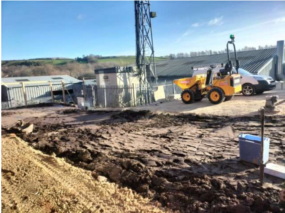
View south-east across rear garden areas from Plot 4 towards Plot 6. Turf remains to be laid.
