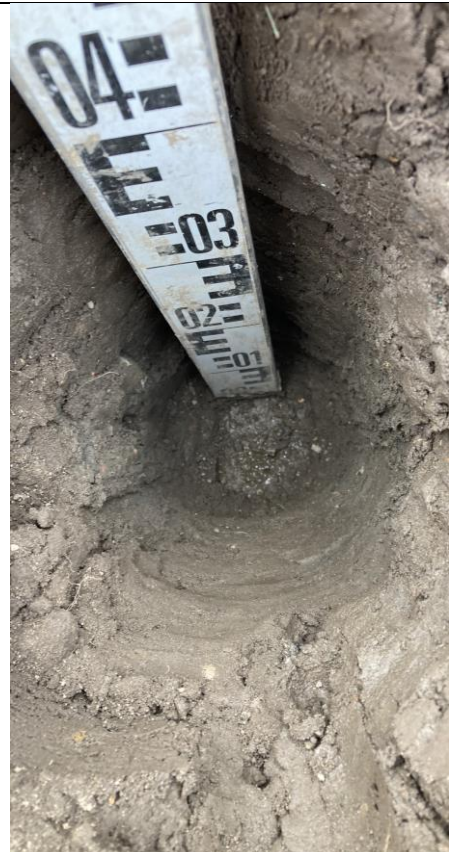
Plot 42: Internal View of excavation
