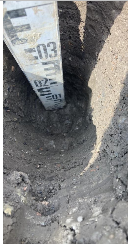
Plot 30: Internal View of excavation
