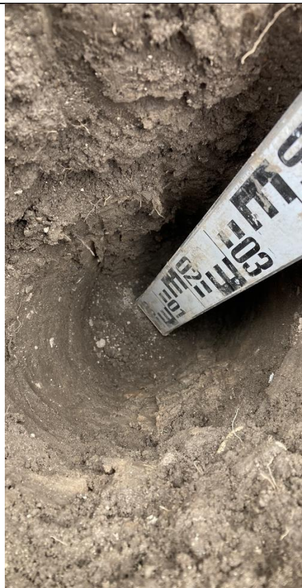
Plot 38: Internal View of excavation
