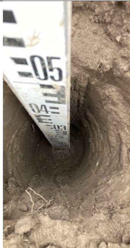
Plot 41: Internal View of excavation
