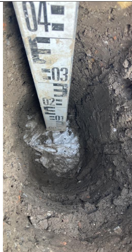
Plot 26: Internal View of excavation
