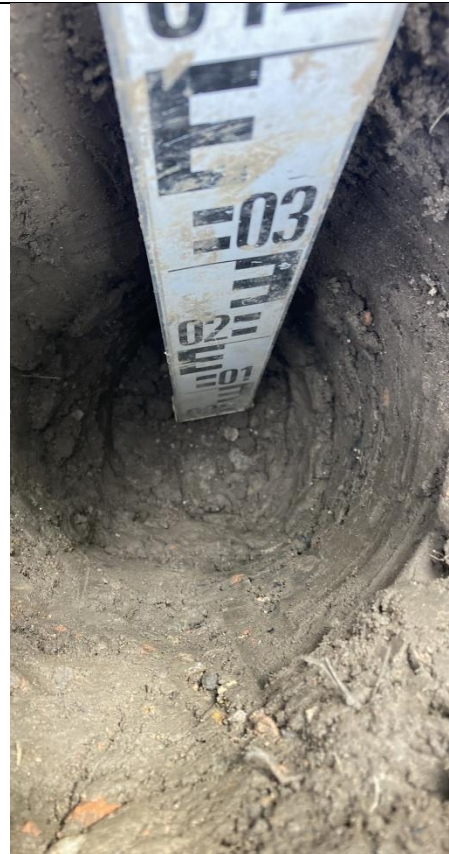
Plot 29: Internal View of excavation
