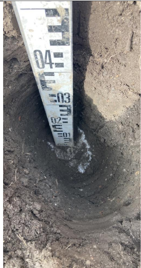
Plot 27: Internal View of excavation
