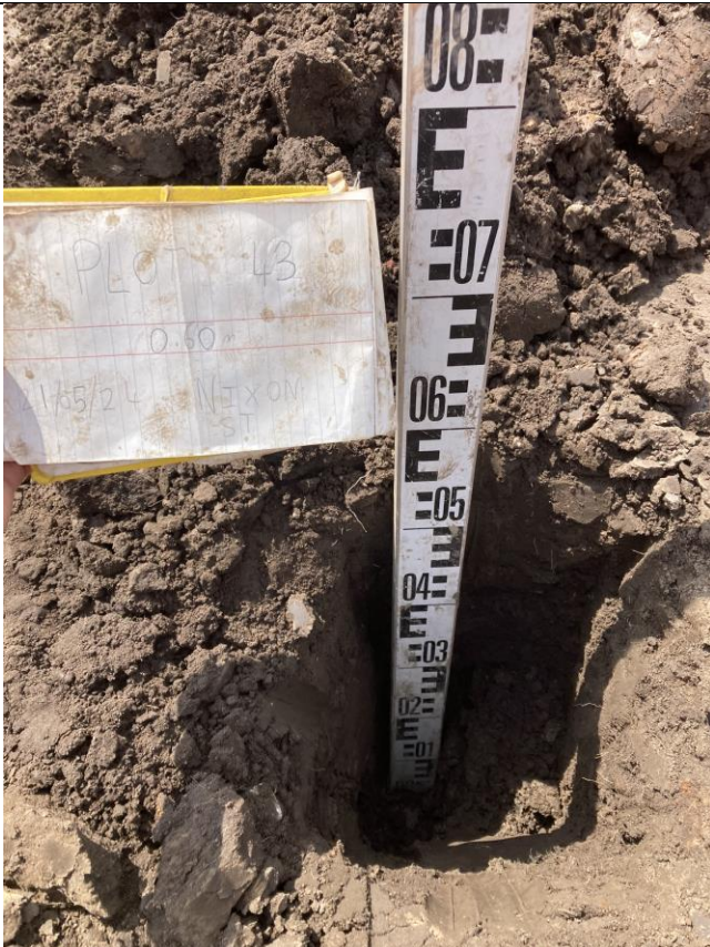
Plot 43: Overview of excavation
