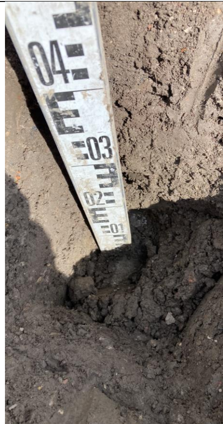
Plot 44: Internal View of excavation
