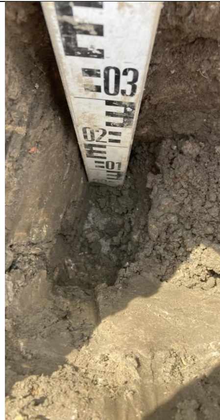
Plot 43: Internal View of excavation
