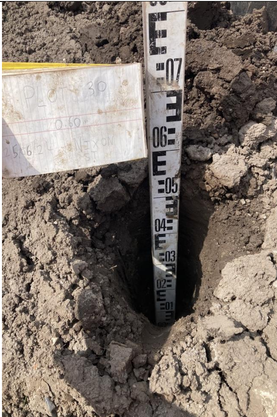
Plot 30: Overview of excavation
