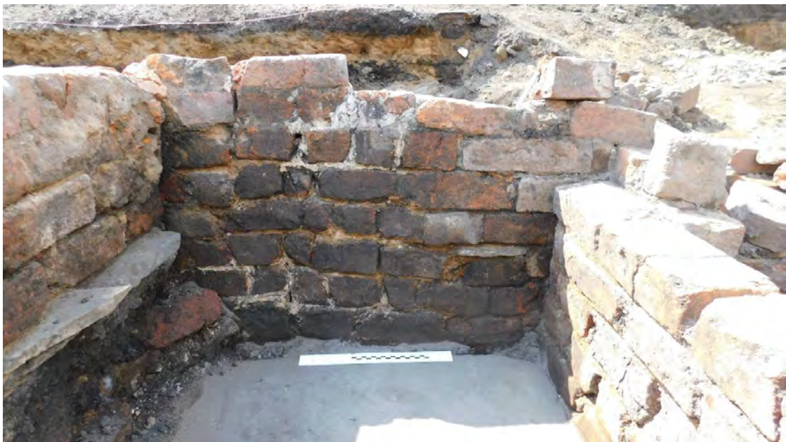
Plate 15: part of western wall of Building 1, looking west
