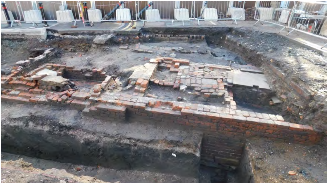
Plate 14: late 18th/ early 19 th -century boundary wall [1006]/[1018] with later structures behind, looking east
