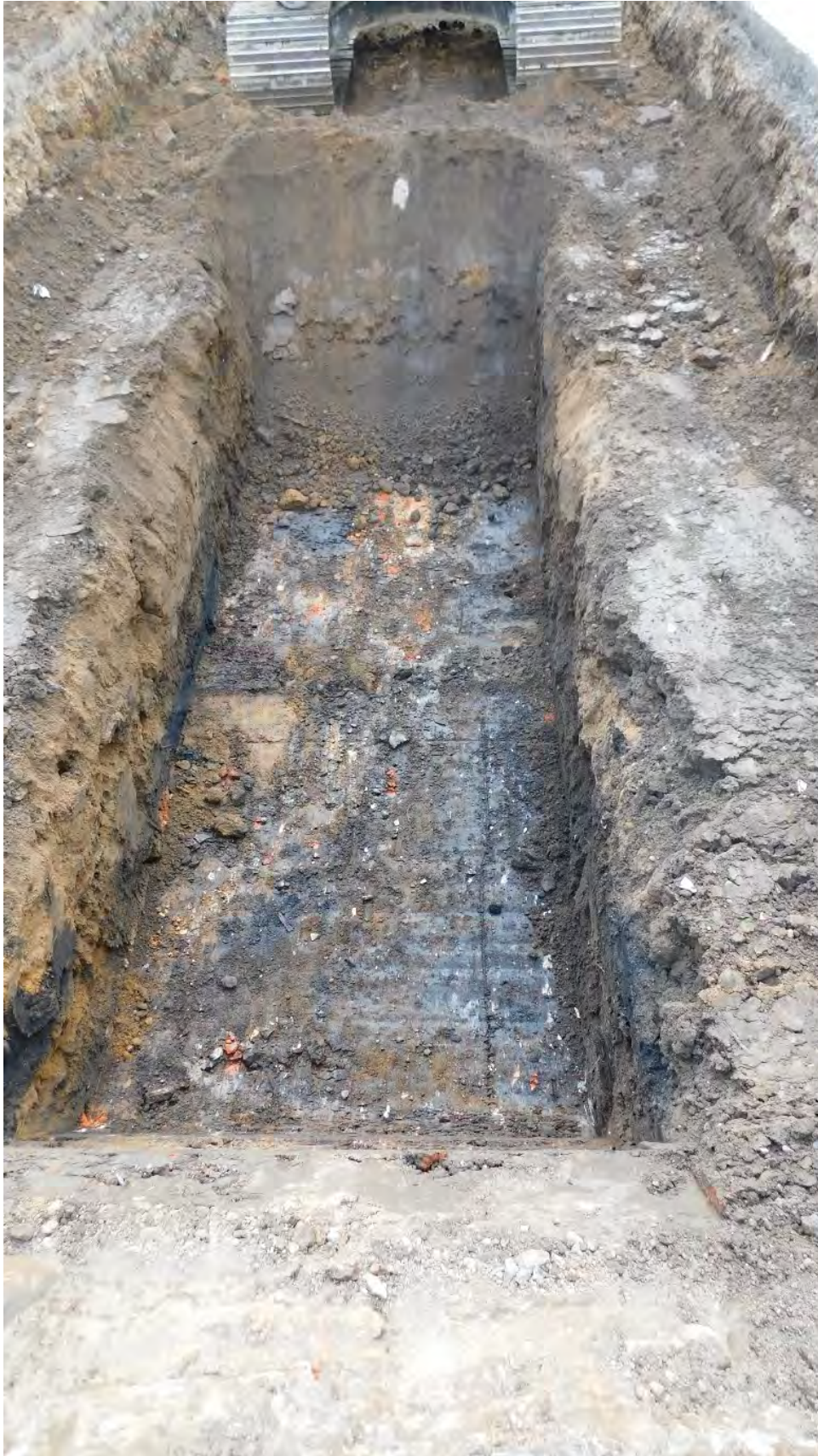
Plate 17: slot excavated in north part of Area B with possible remains of floor surface at base, looking south
