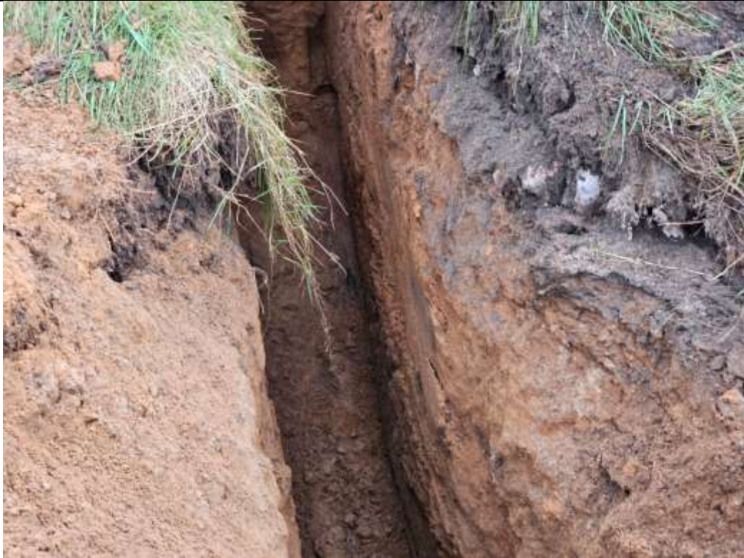
Trial Pit S2 – after excavations
