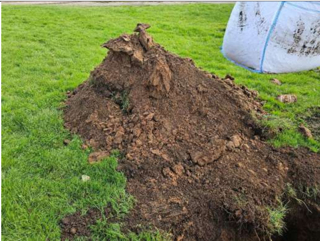
Trial Pit S6 – excavated spoil
