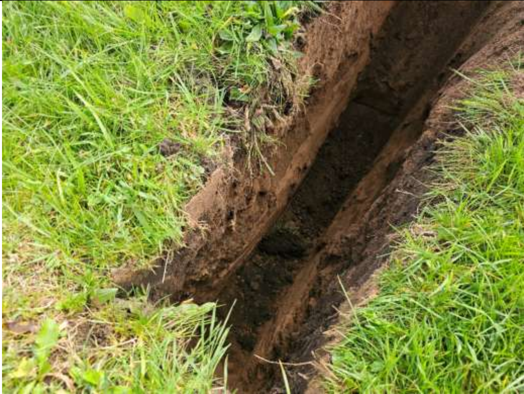
Trial Pit S5 – after excavations
