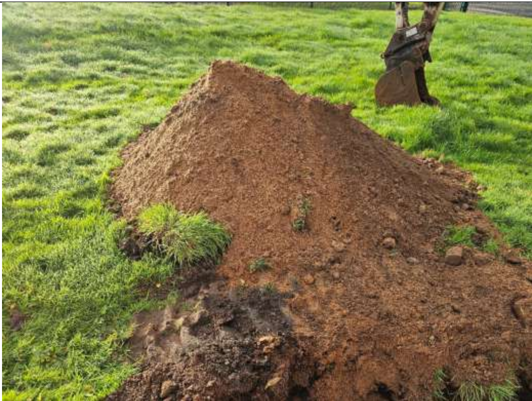
Trial Pit S4 – excavated spoil
