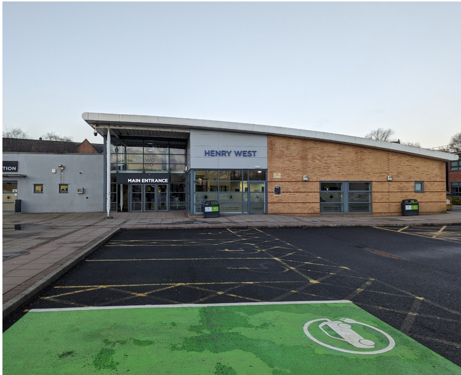
5 View towards the Henry West building from the main car park
