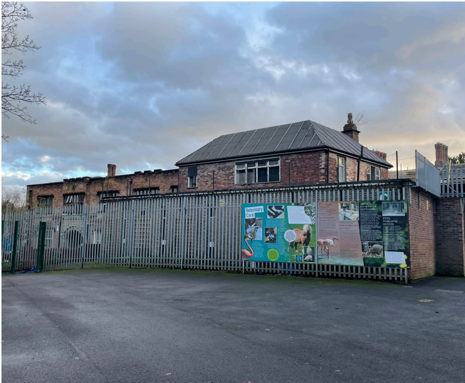
4 View towards Hopwood Hall from the Animal Management facilities
