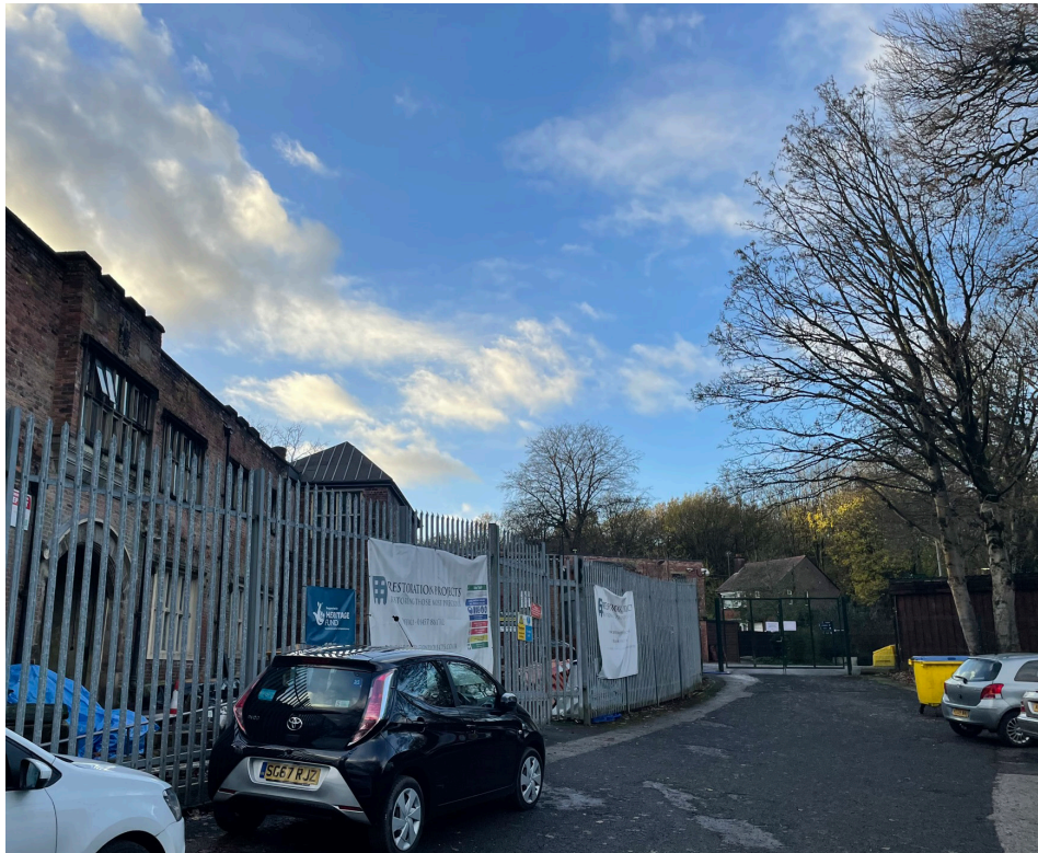
5 View towards the main entrance to Hopwood Hall from existing access road
