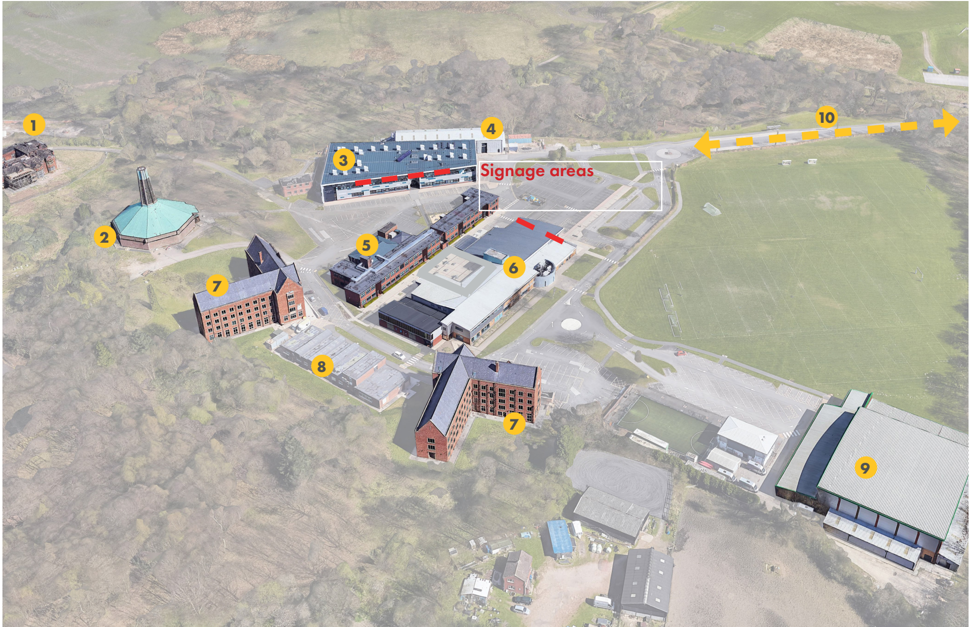
Existing Aerial View
