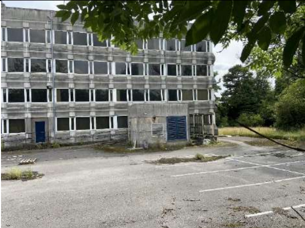
P5: Looking at north-west corner of the building.
