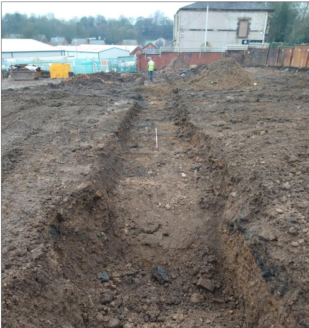
Plate 6: A post-excitation view along Trench 2, revealing some initial remediation and natural ground. Looking west.
