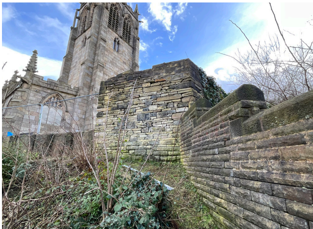
2.05 Junction between Partnership House boundary wall and Grade II listed Wall to the North West of Church of Saint Chad (seen to left of image)
