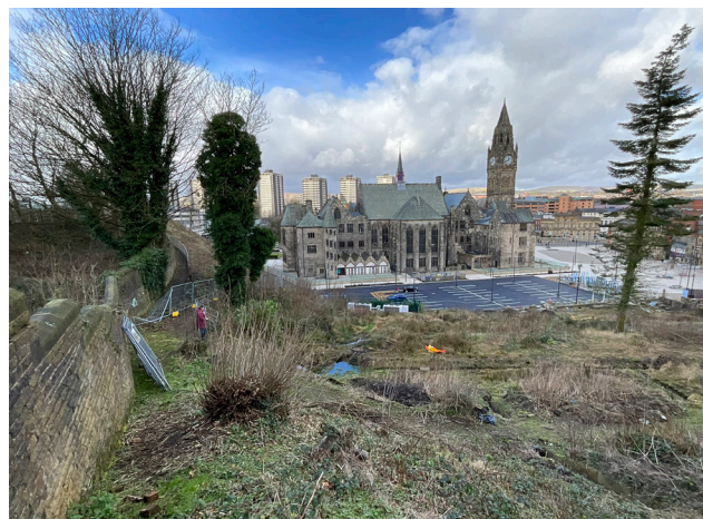
2.06 View from top of boundary wall looking north back towards Rochdale Town Hall and over Broadfield Park Slopes
