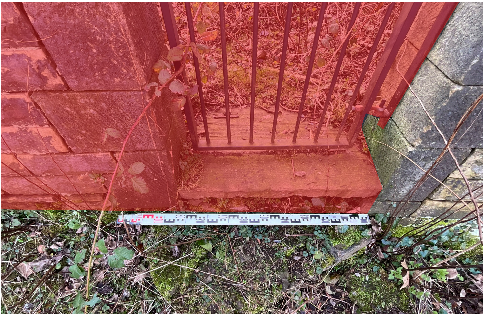
4.05 Plan view showing pedestrian gate opening, with measure stick at base reading 1 metre
