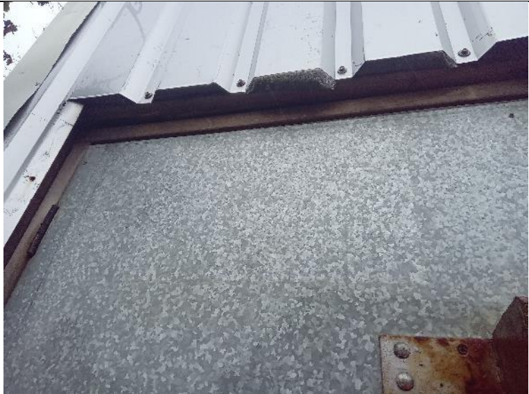
Figure 13. Metal cladding infilled.
