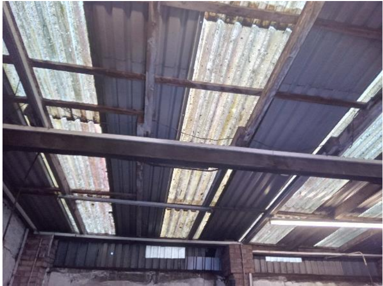
Figure 18. Metal sheet roofing and skylights.
