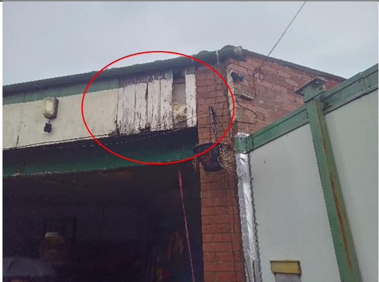
Figure 9. Missing panelling.
