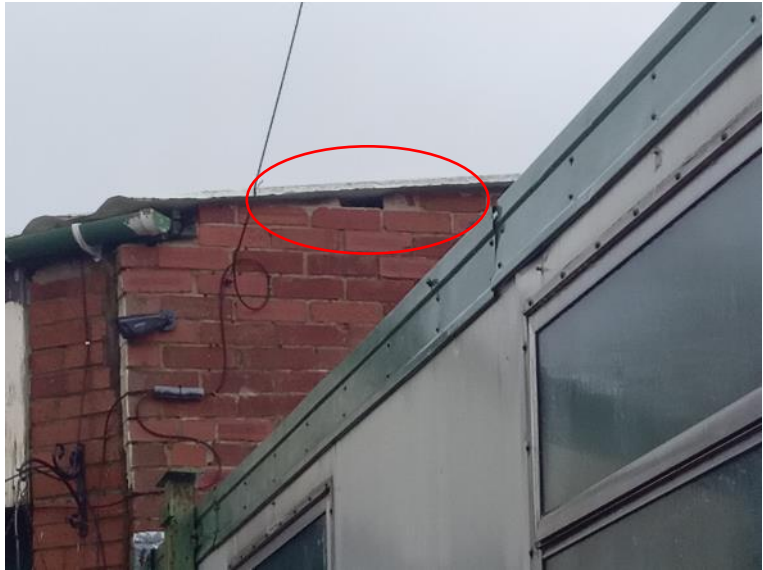
Figure 10. Missing brickwork/mortar.
