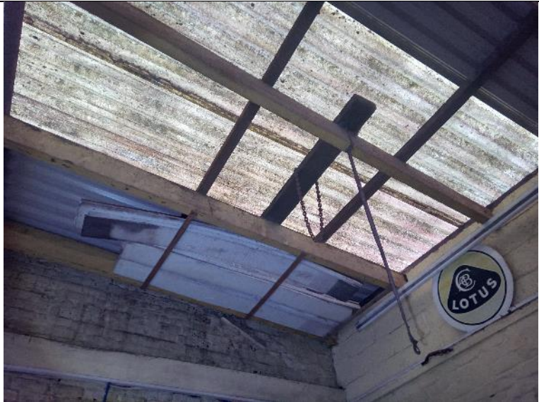
Figure 21. Metal sheet roofing and skylights.
