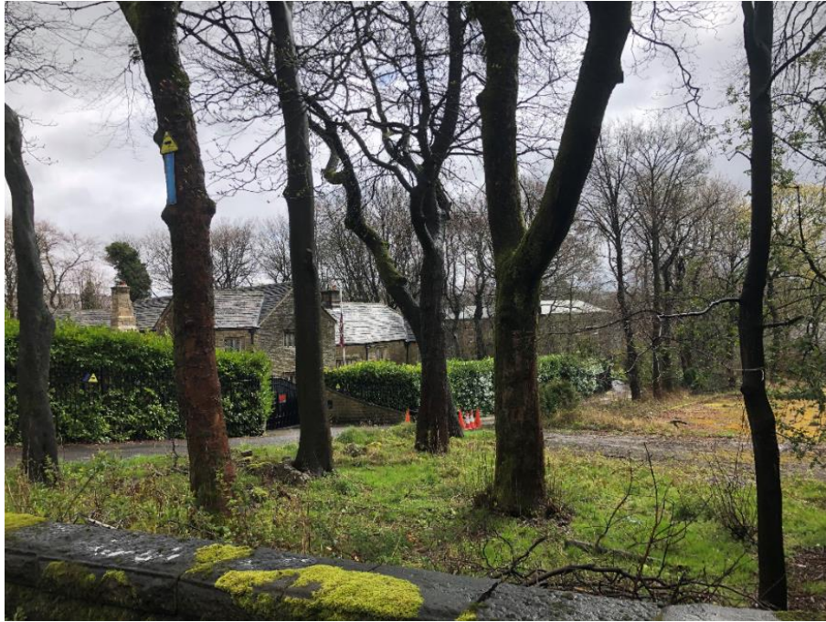
Figure 4.1: Stubley Old Hall, west (front) elevation
