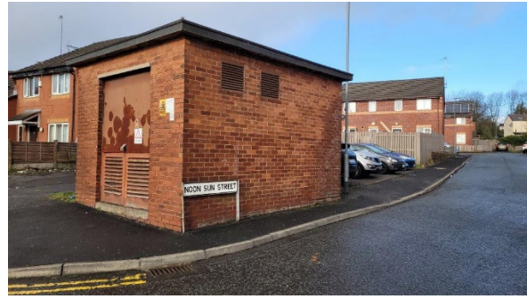
Block C – Sub Station with Site Beyond
