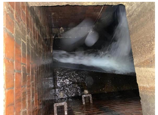
BOTTOM CHAMBER DROPSHAFT AND OUTLET
