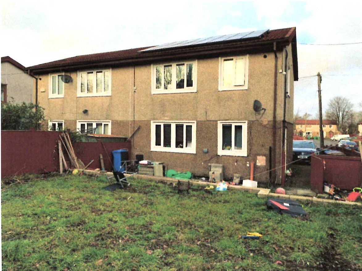
Rear elevation of 96 Waithlands Road
