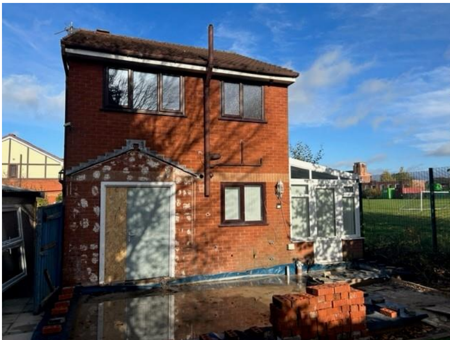
Rear view of property showing previous rear conservatory removed.
