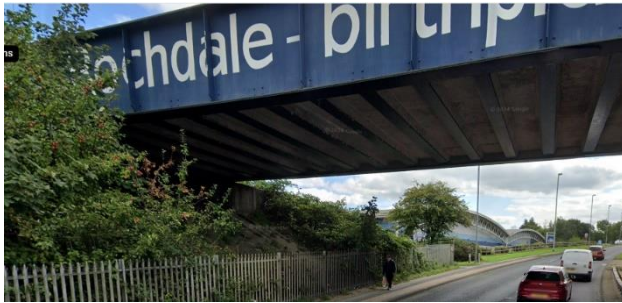
Figure 3A: Rochdale Bypass (A664)
