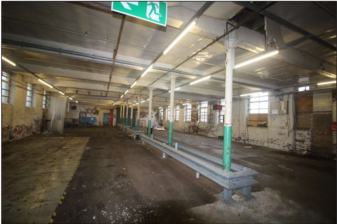
Plate 10: The ground-floor of the c.1890-1908 shed fronting Hill Street, facing north
