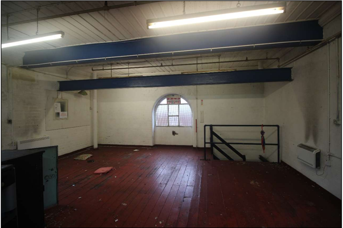
Plate 16: General view of the first floor to the engine house, facing west
