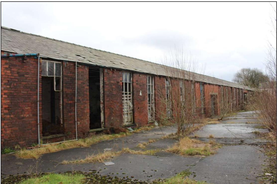
Plate 5: General view of the western elevation to the ropery, facing south-east
