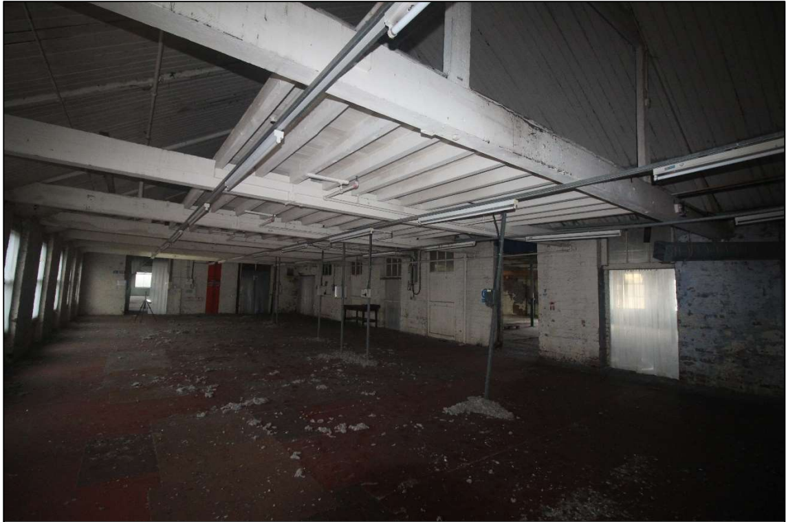
Plate 14: General view of the second floor of the original warehouse, facing east
