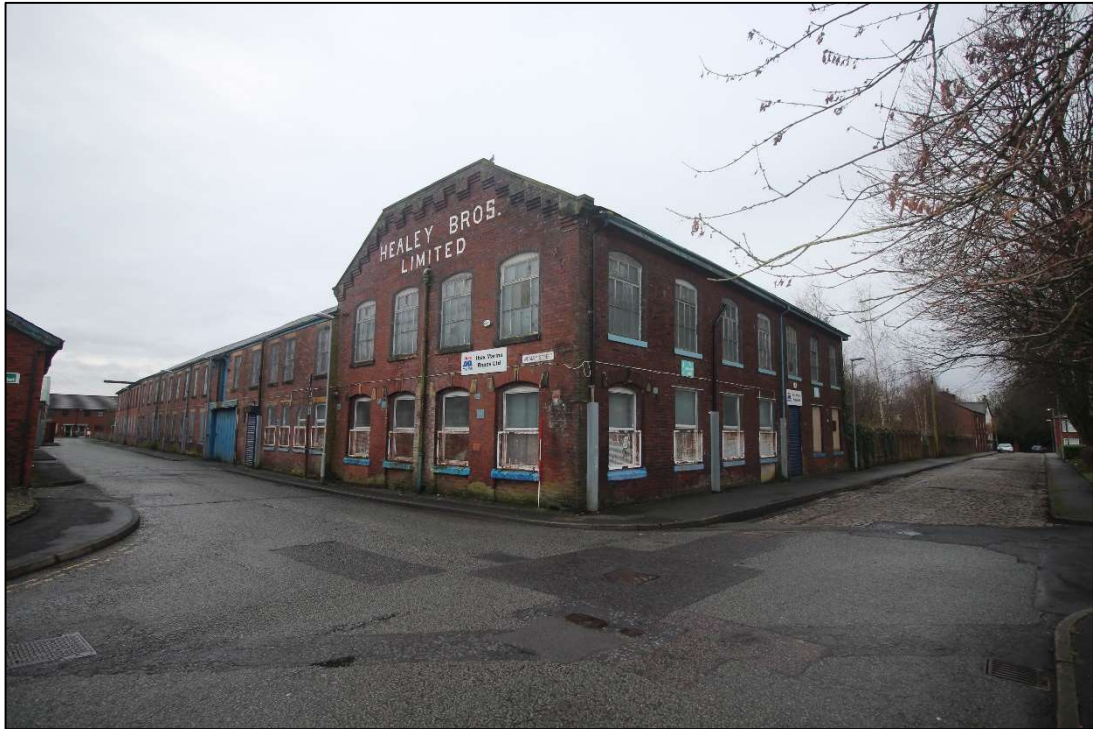
Plate 2: General view of Marina Works, facing south-east
