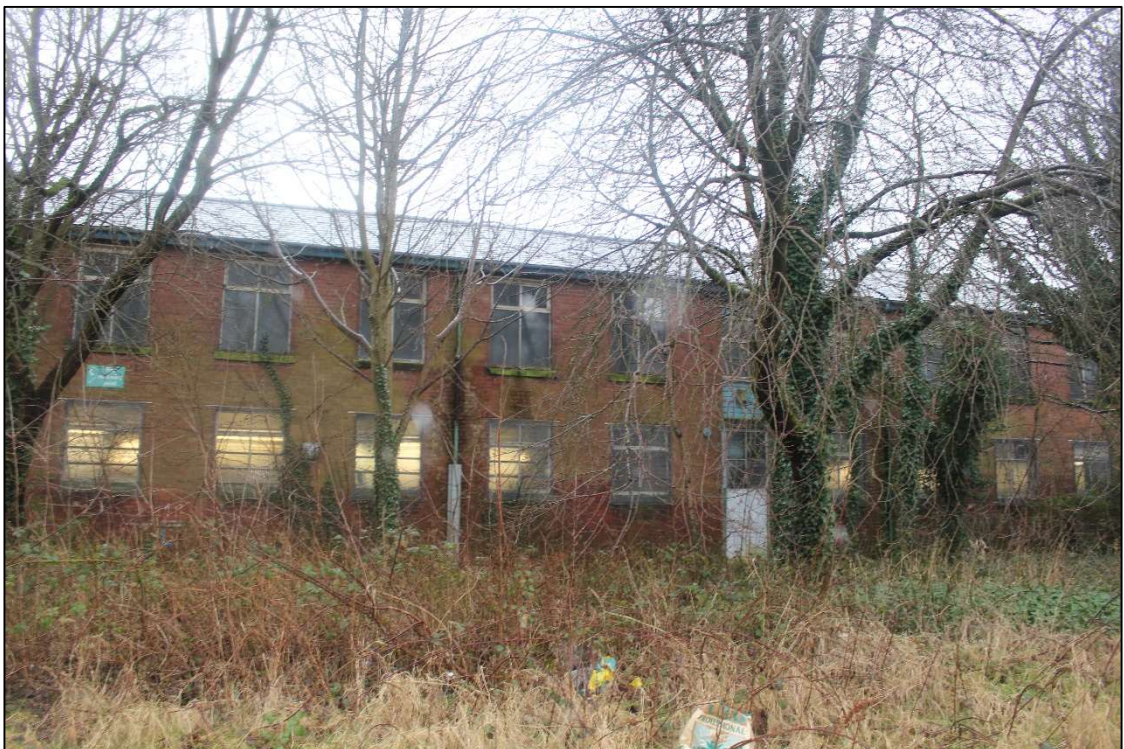
Plate 7: Western elevation of the c.1890-1908 building fronting Hill Street, facing west
