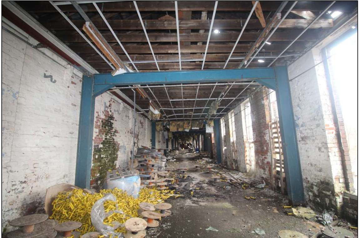
Plate 8: Internal view of the original ropery, facing south
