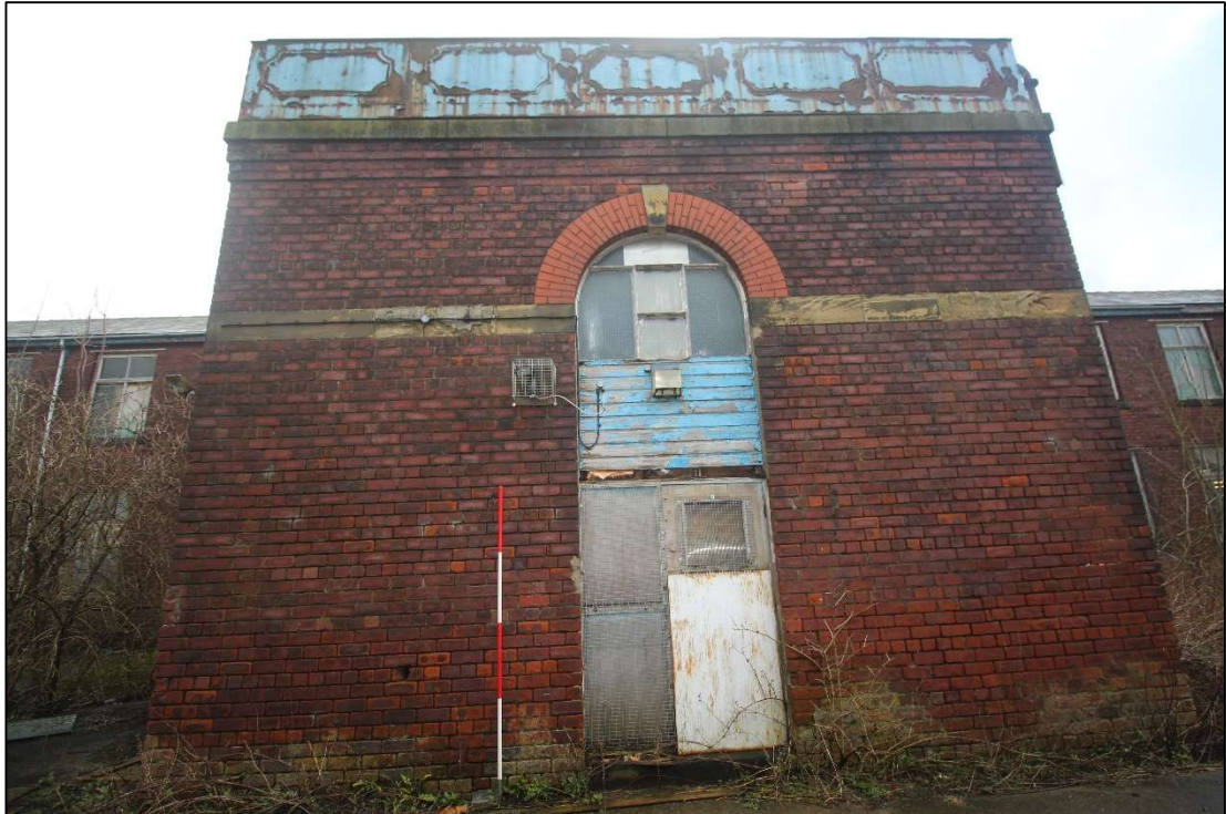
Plate 6: Western elevation of the engine house, facing east
