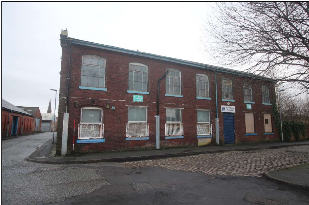
Plate 3: The western elevation of the office building fronting Brunswick Street, facing east
