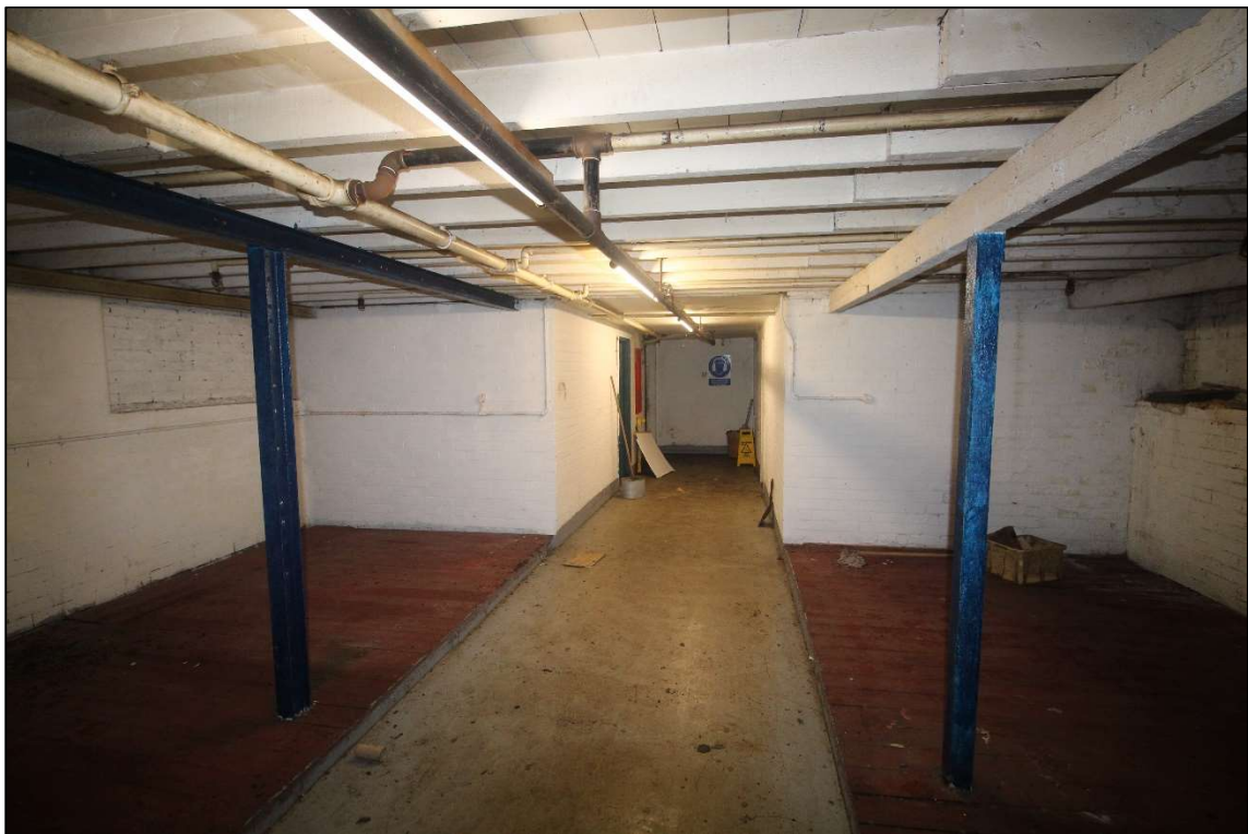
Plate 15: General view of the ground floor to the engine house, facing south
