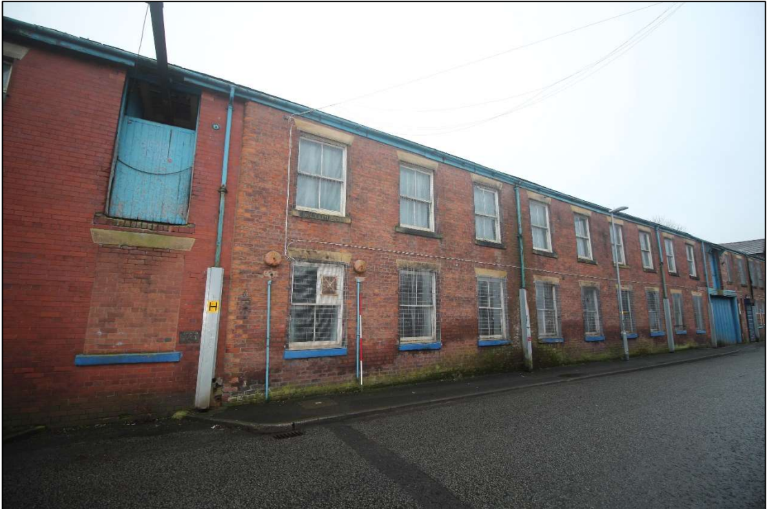
Plate 4: General view of the original 1850 warehouse fronting Wesley Street, facing south-west
