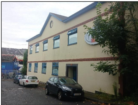
Figure 2.2: View of the east elevation of the building (Cheetham Street).
