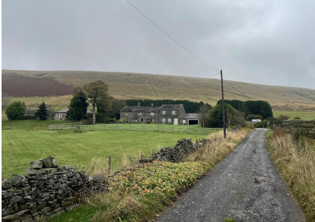
Figure 4.6: View of Fecit Farmhouse with attached stable and shippon from the south west on Fecit Lane
