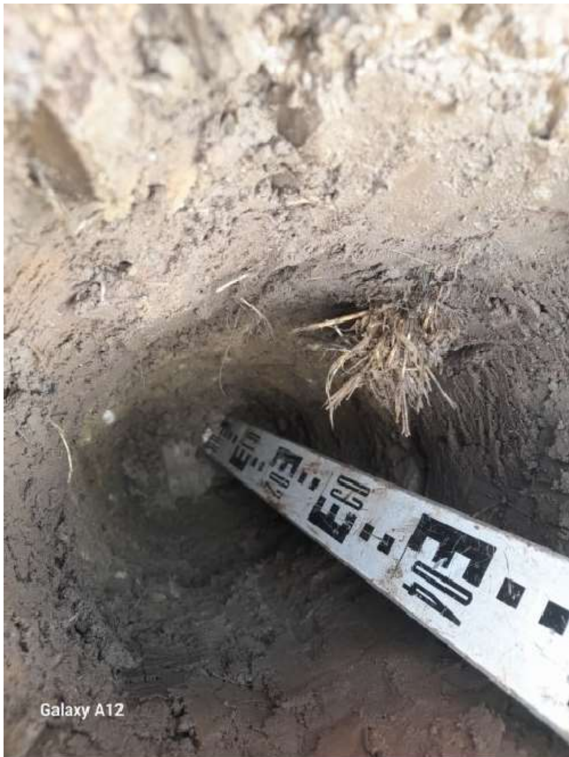
Geotextile at the base of HDP3.
