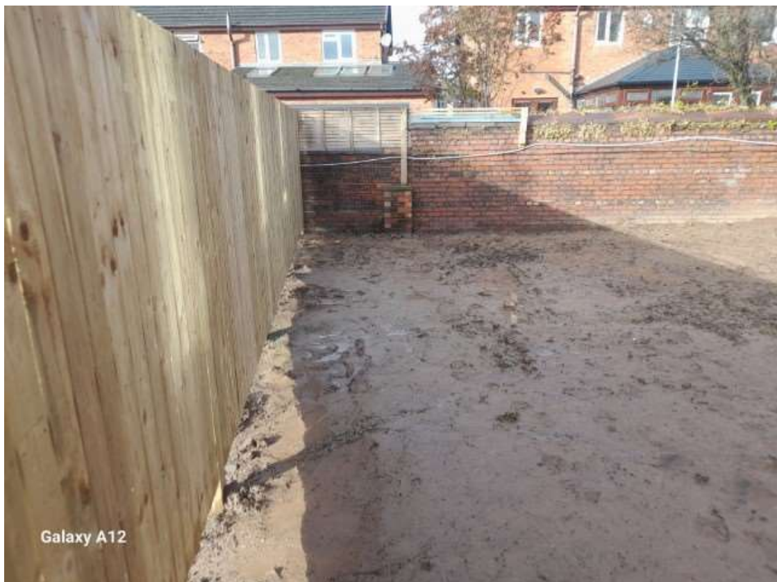
View west along southern boundary of Plot 1.
