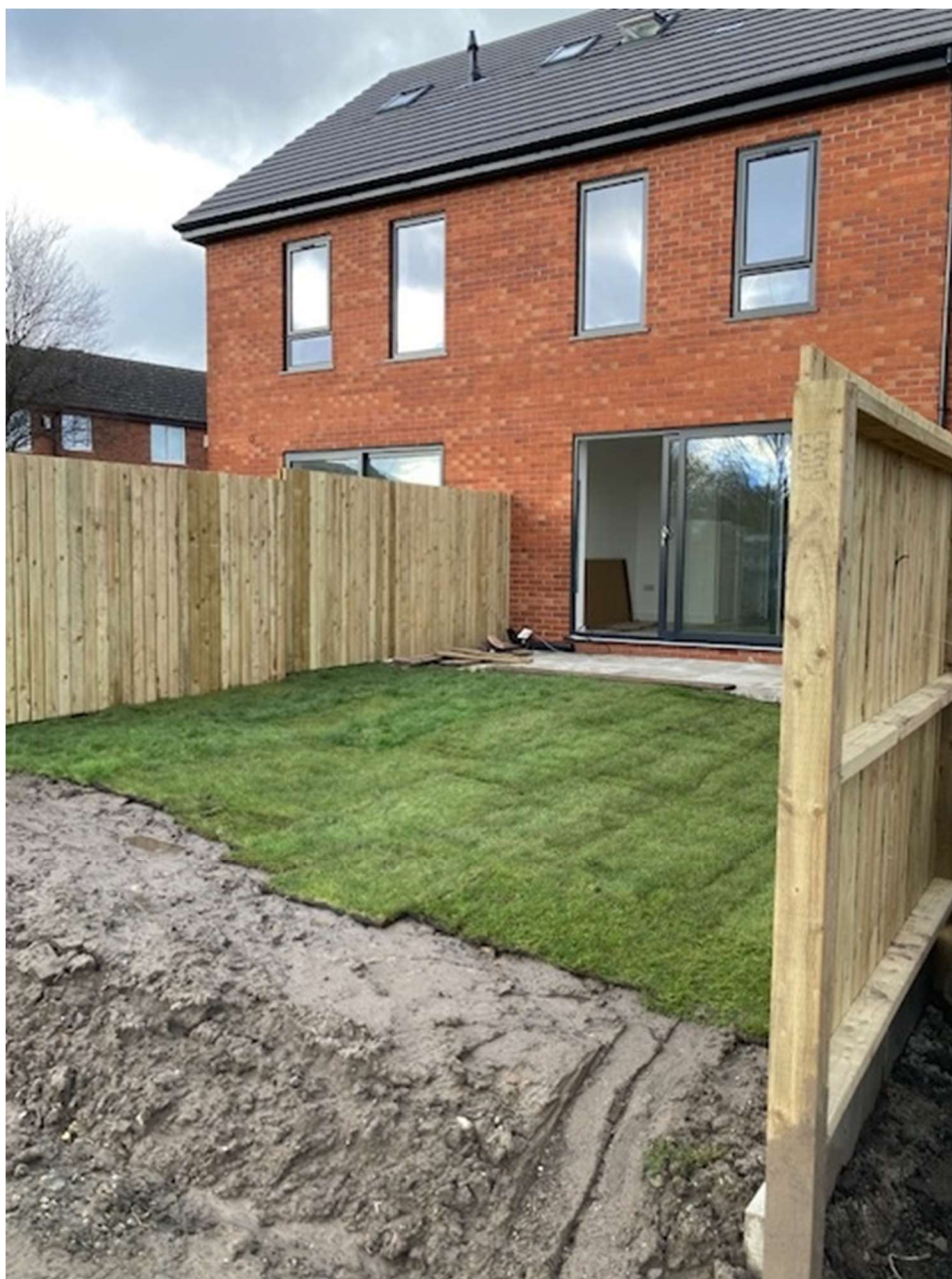
View north-west across the garden area of Plot 2, following placement of turf.
