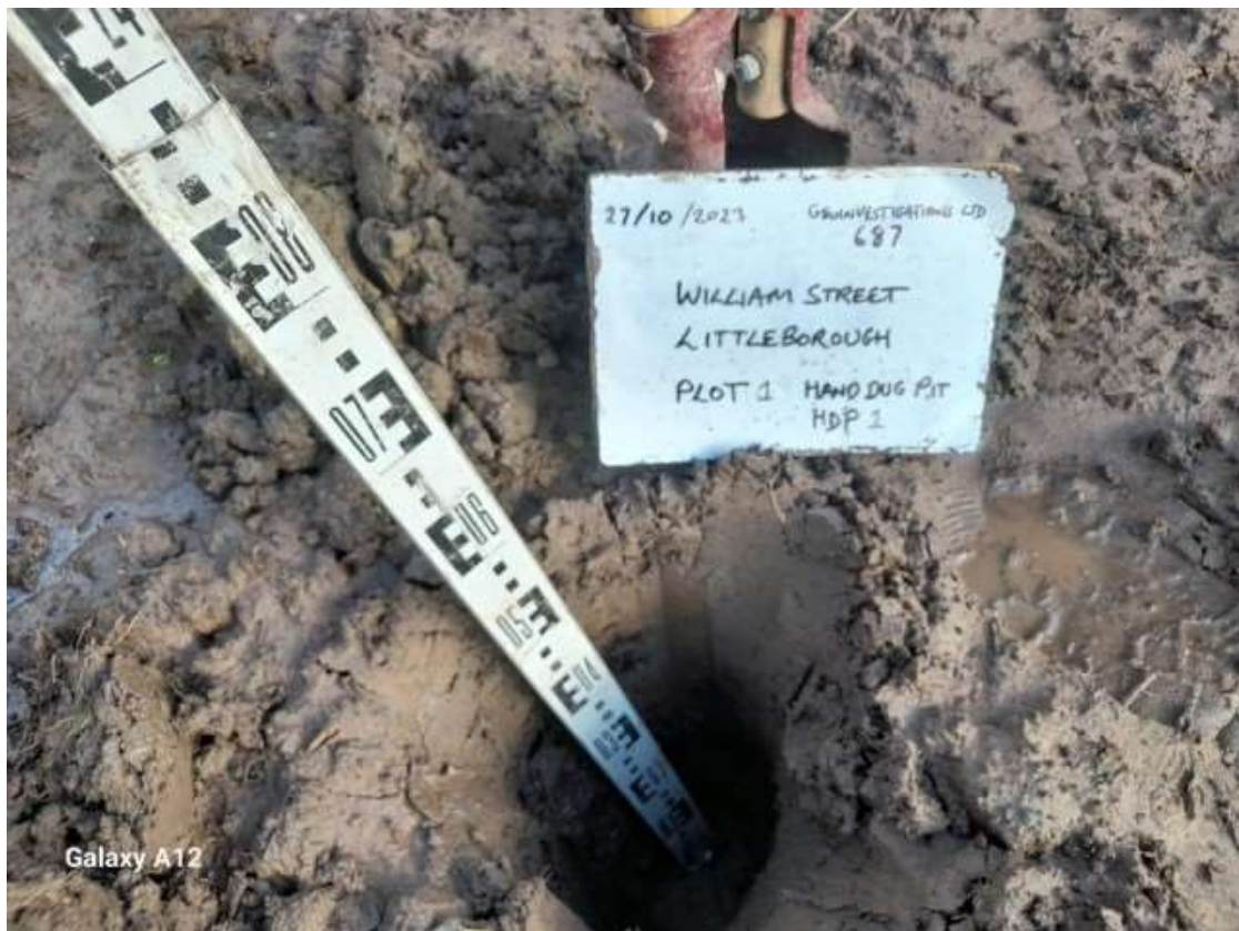
Hand dug pit HDP1 (Plot 1).
