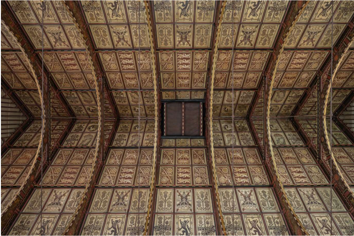
Images of the Great Hall ceiling panels with protective netting installed underneath taken at ground level.
