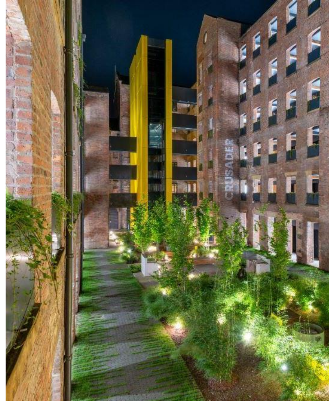
CRUSADER MILL, MANCHESTER CITY CENTRE
