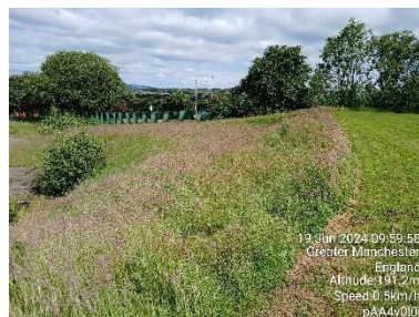
Embankment in the west of the site
