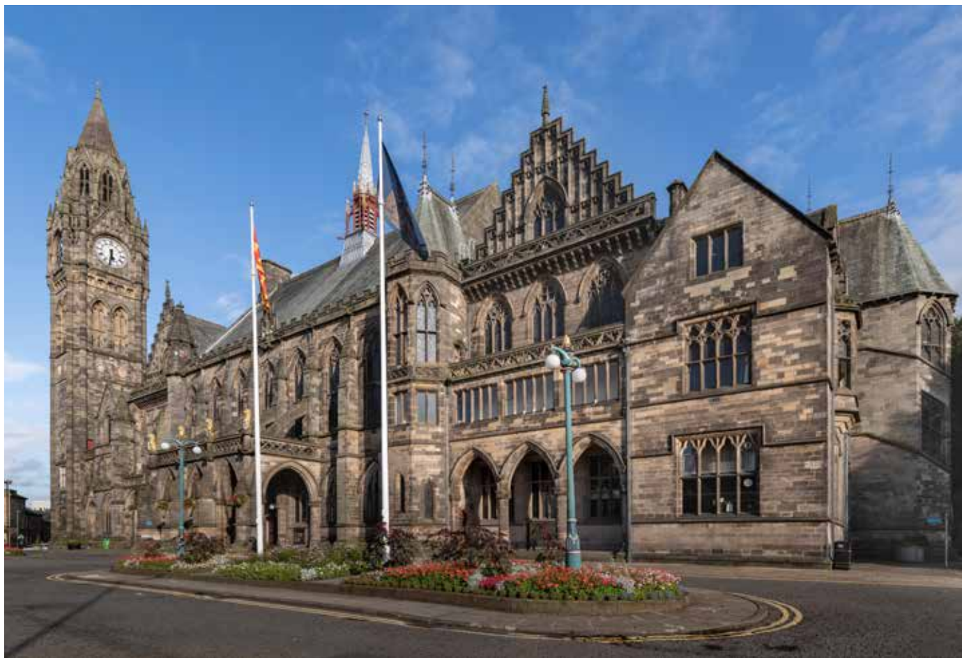
2.1 The north front (Damian Griffiths 2019)
