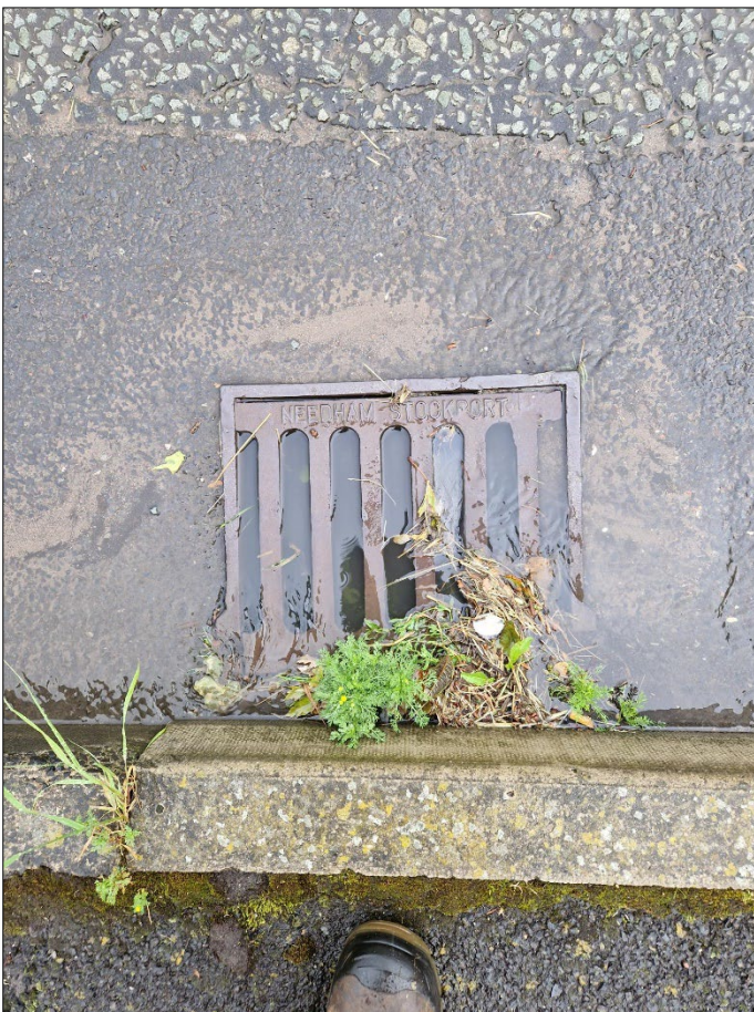
Road Gully Condition Example
