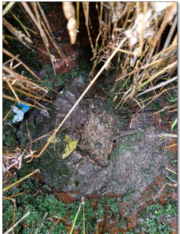
MH3 Internal View Before Clearing
