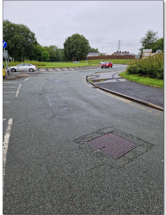
Manhole S8 Location View
