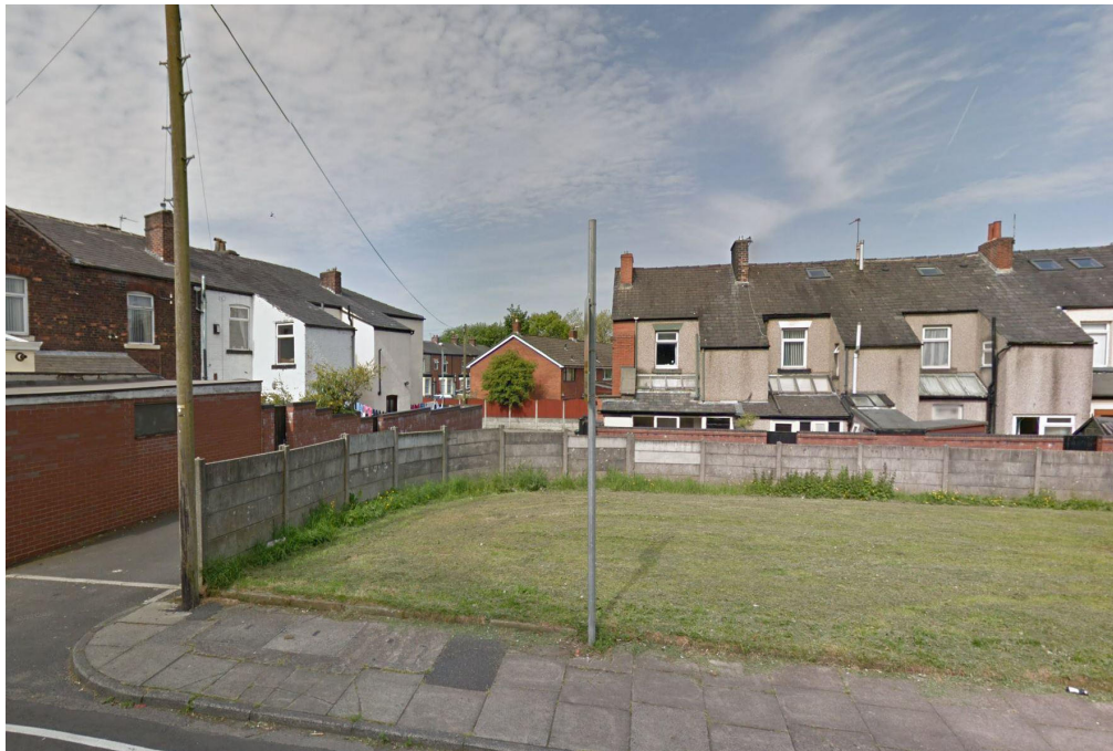
Existing boundary treatment around the site and brick wall with gate access securing the terraces to the rear.
