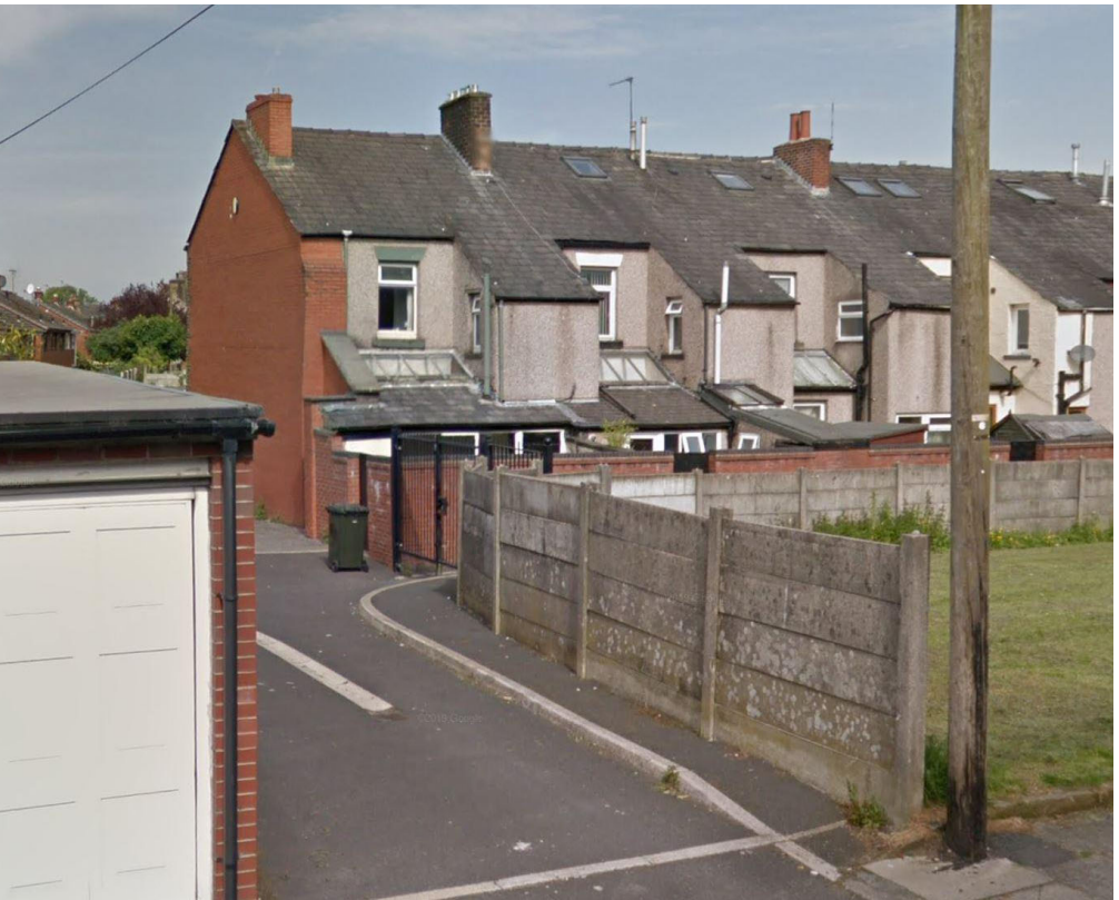
Existing metal railings with gate securing access to alley.
