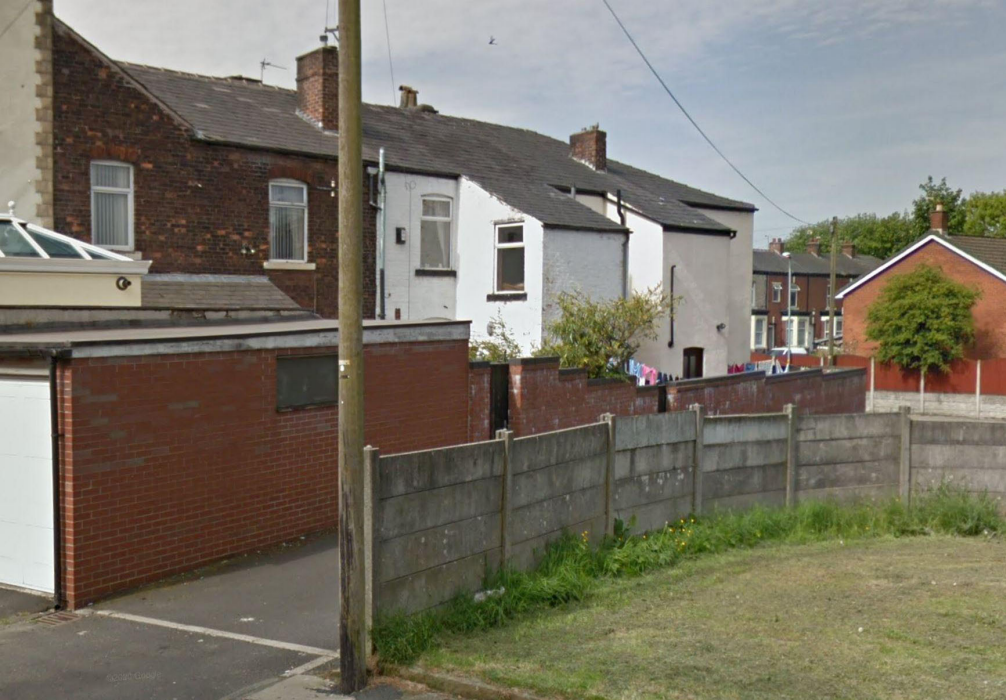
Red brick wall with rear gate access securing neighbouring properties.
