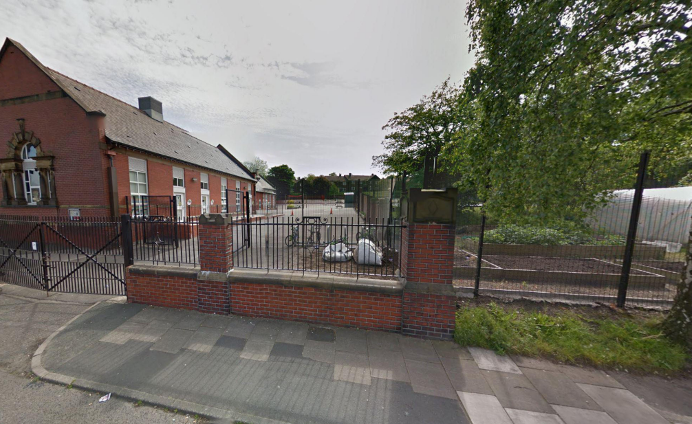
Existing brick wall with railings securing the primary school opposite the site.
