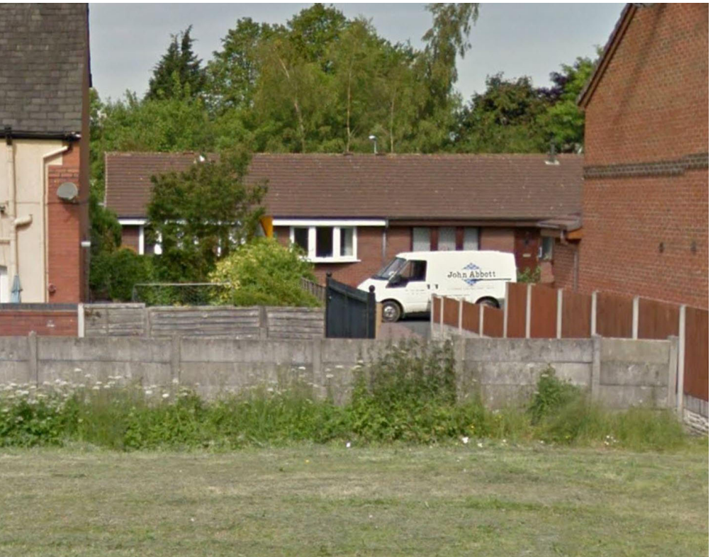
Existing railings with gate access securing the alley. Timber panel fencing with concrete posts along boundary line.
