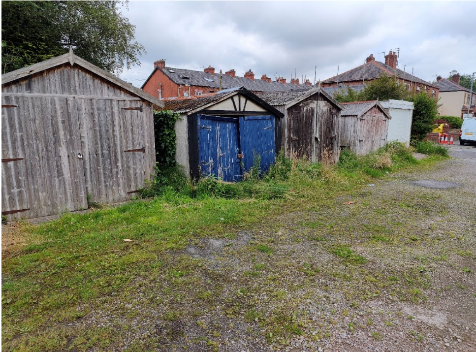
Photograph 3: Garages in the west of the Site (in relatively poor condition), facing northwest.
