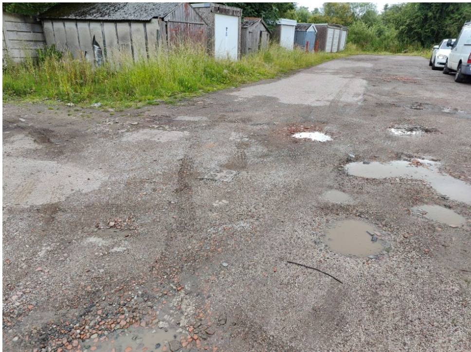
Photograph 6: Western-central area of the Site - several of the existing garages can be observed surrounded by overgrown vegetation.
