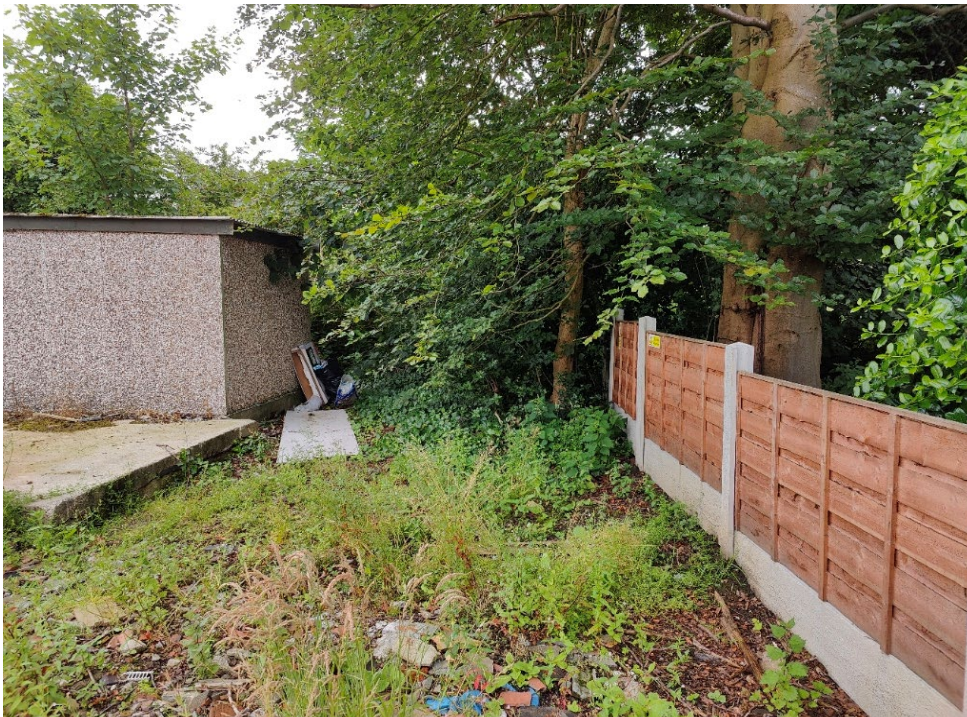
Photograph 10: A garage in relatively good condition and soft standing along the southern boundary of the Site, looking east.
