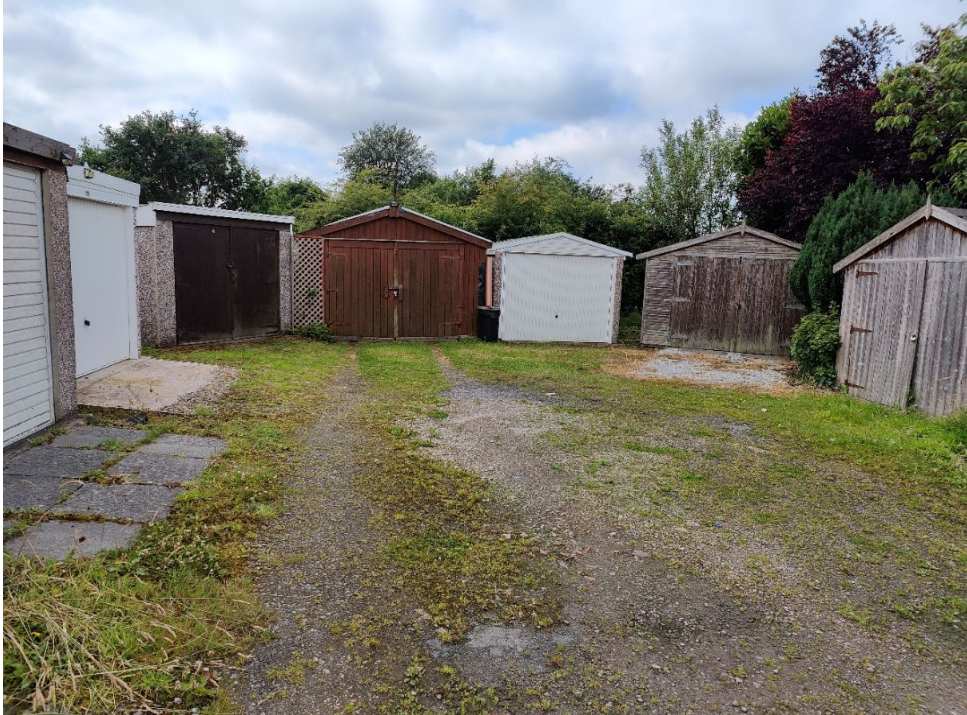
Photograph 1: Several garages in various stages of disuse on Site 1, facing south.
