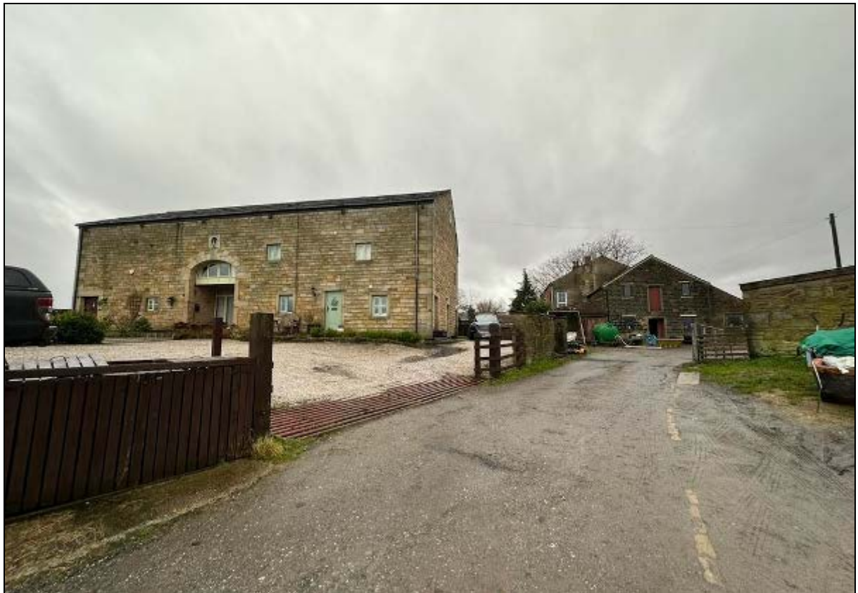
2. The wider site, viewed on approach, with farmhouse in centre distance
