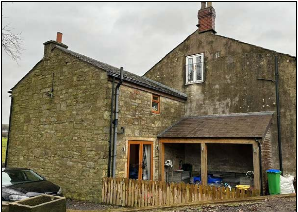
6. Rear elevation of the cottage and adjoining store
