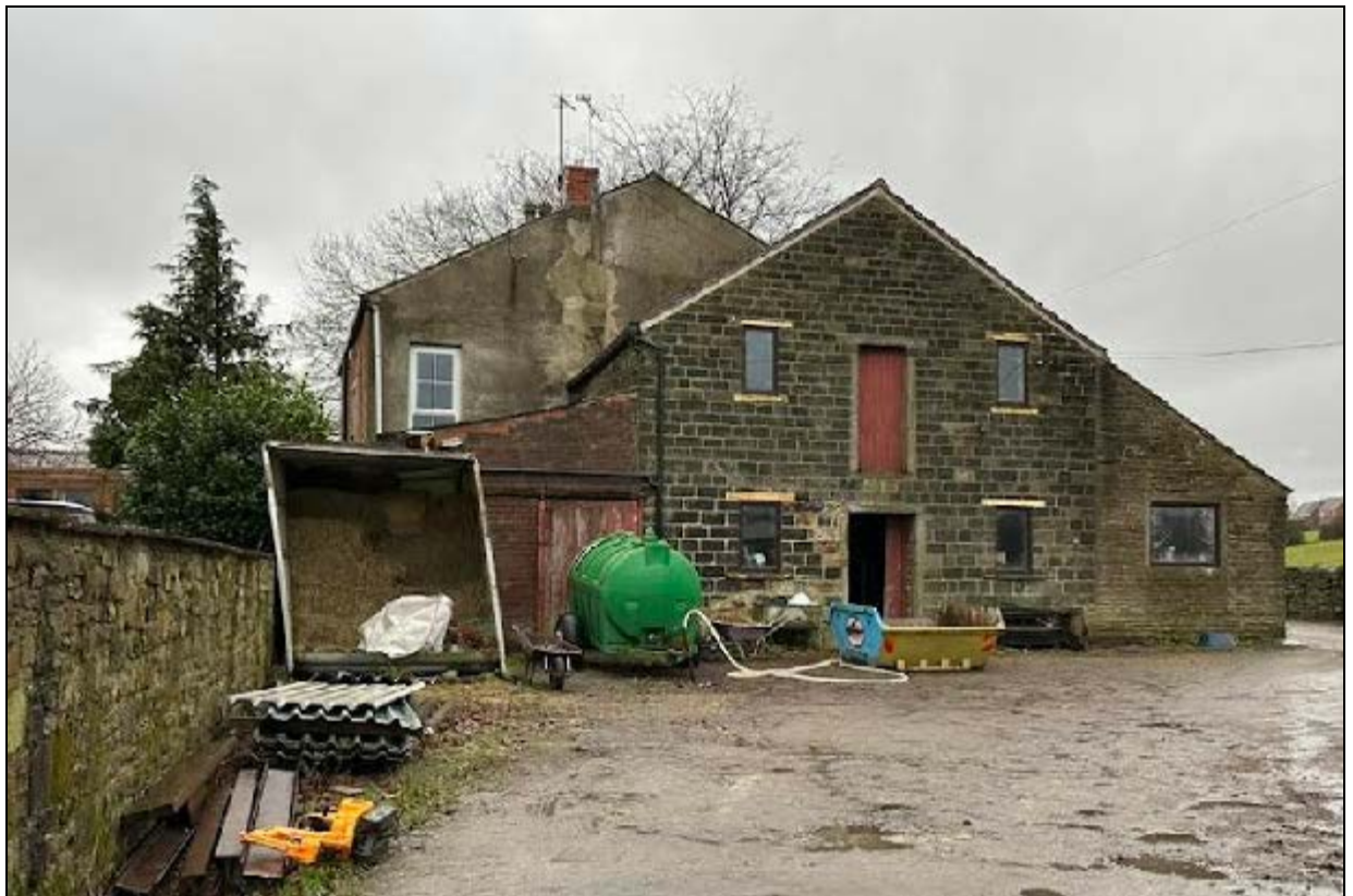
5. East side elevation, showing stable attached to the house
