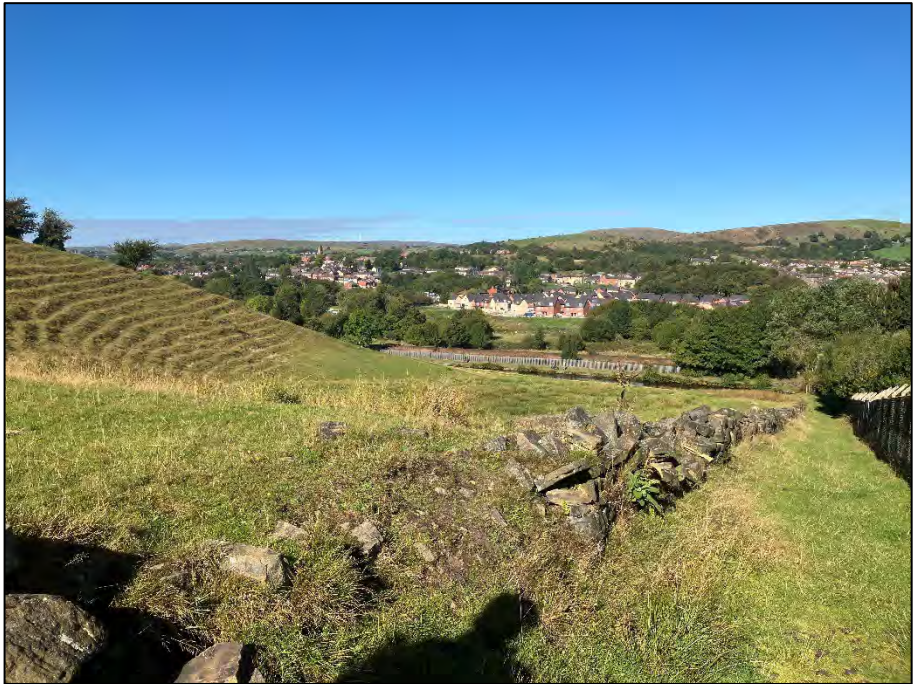
Photograph 6: View of site looking northwest towards the Rochdale Canal. Area of 'Landslip' is on the left of photo and boundary with Akzo Nobel site is on the right.
