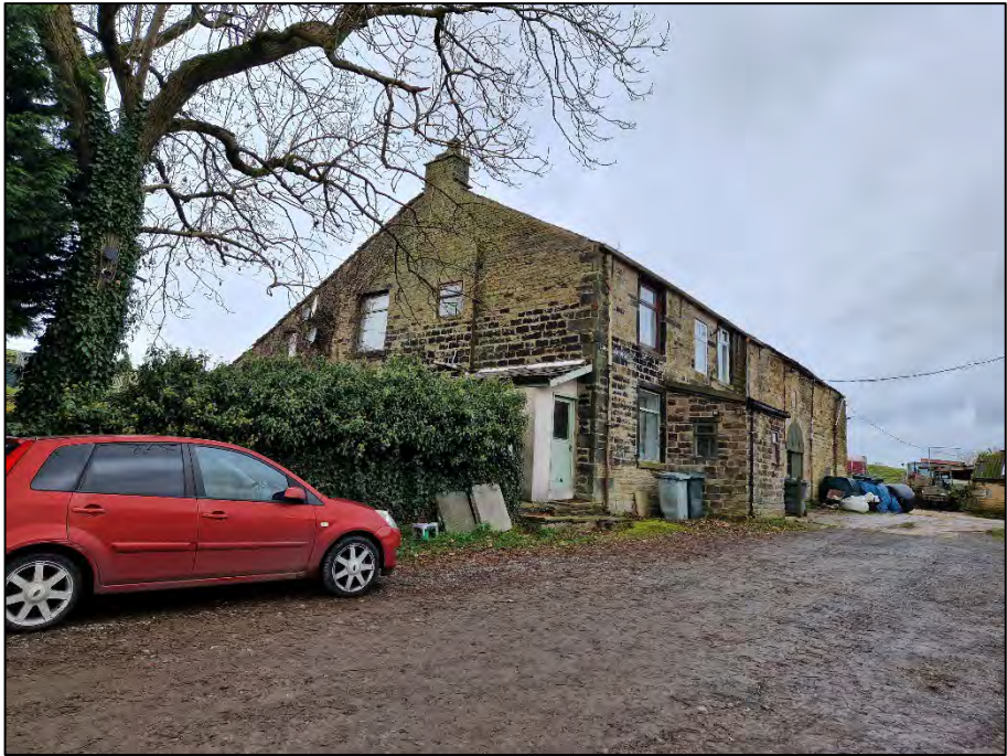
Photograph 3: Residential Buildings at Lower Cleggswood Farm (heating oil tank in right of photo).
