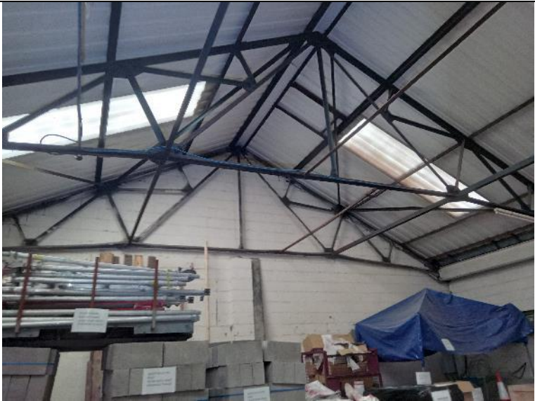
Figure 22. View of interior space 2 – facing west.
