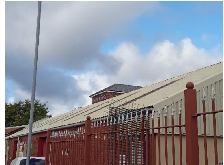
Figure 3. Metallic roofing intact.
