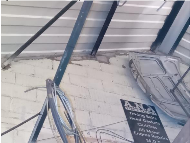
Figure 19. Mortar intact – eastern gable.
