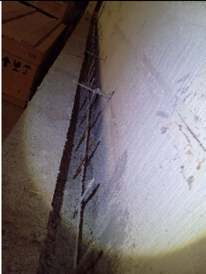
Figure 26. Cavity wall filled with cement.
