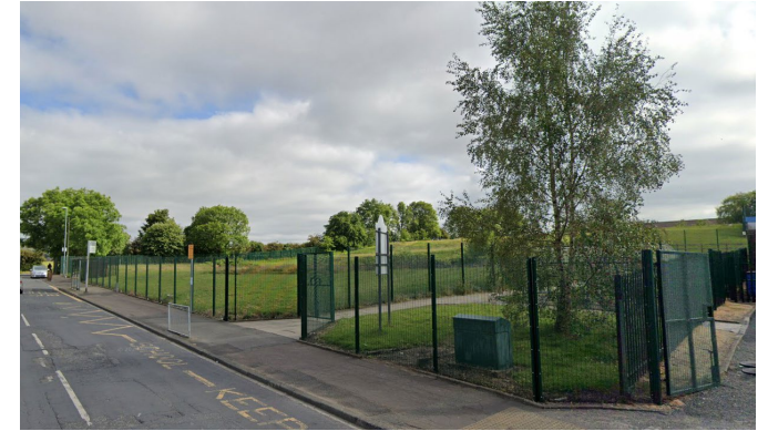
View of site 01 from Sutherland Road
