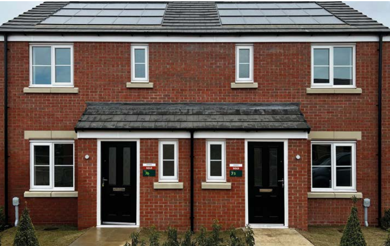
New Build (front and back elevation) - 3.75kWp
