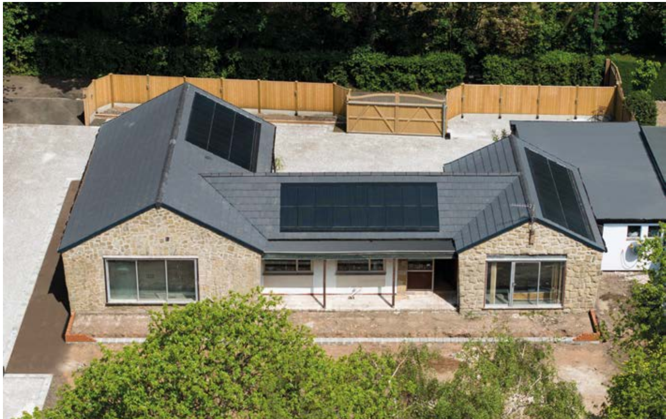
Re-roof (Tiles used - Sandtoft 2020 Antique Slate) - 7.75kWp
