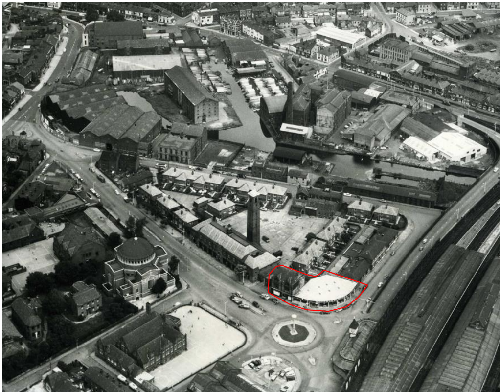
Figure 3.11: 1964 Aerial Photograph of Maclure Road (courtesy of Rochdale Local Studies). The location of the Site is outlined in red.
