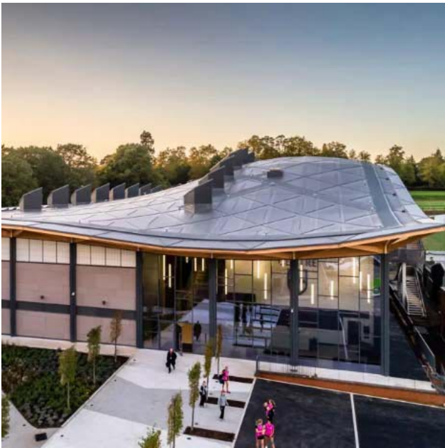
Sika Flat single membrane roof
