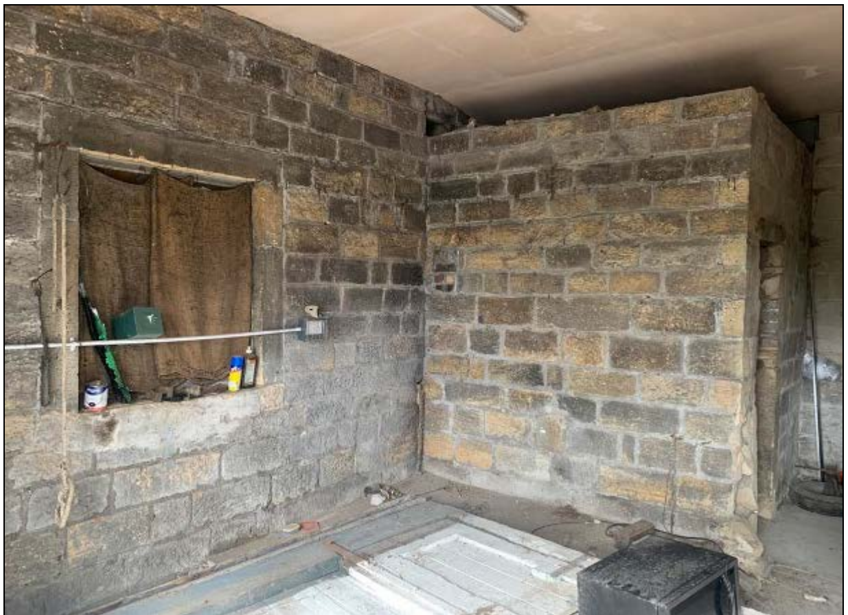
15. Interior of store, showing stable window
