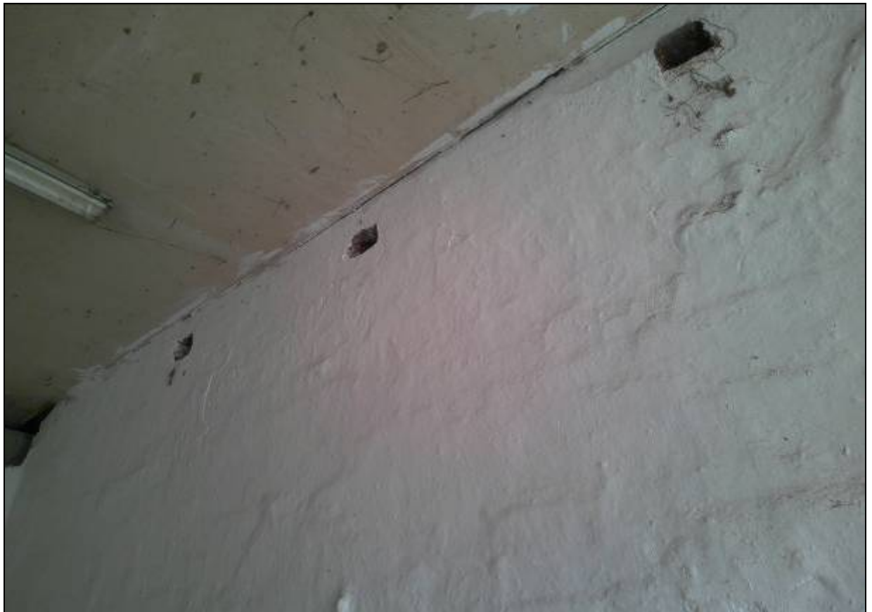
12. Evidence of joists in the shippon, indicating it was originally lofted
