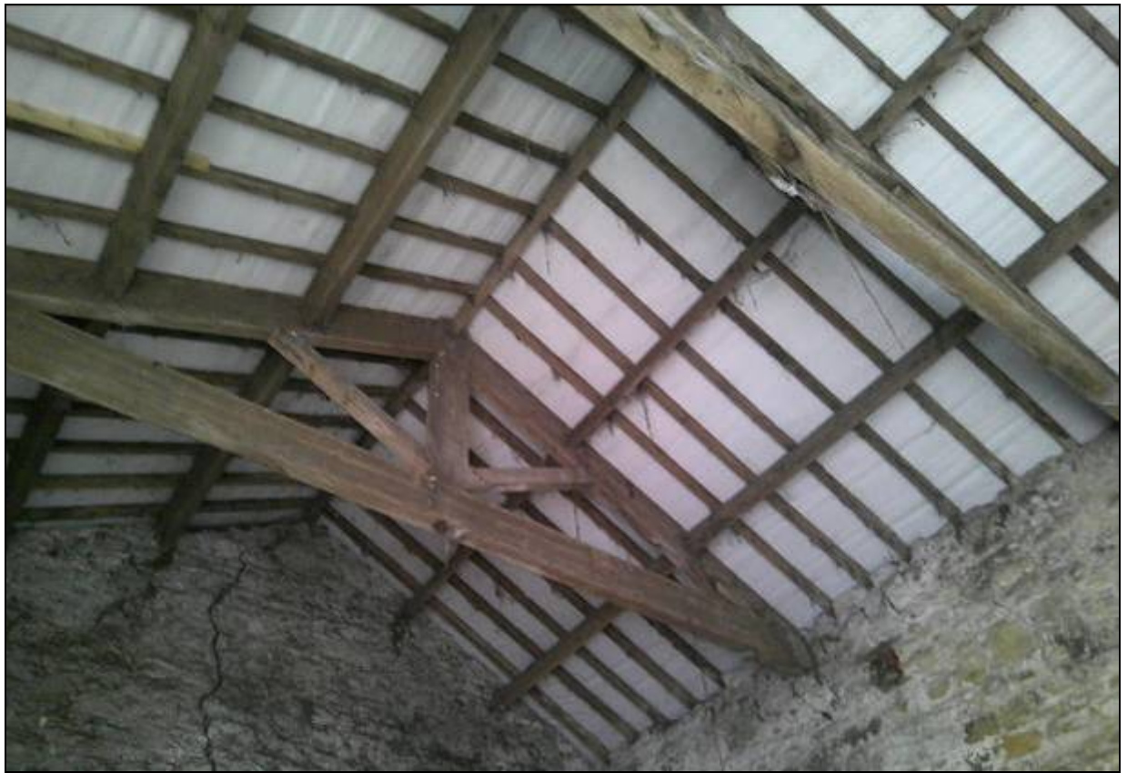
8. Kingpost roof trusses of the barn
