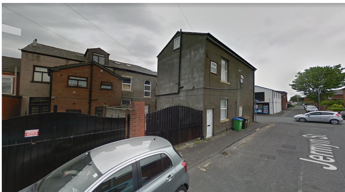
Photo above shows the black gates providing access to rear yard taken from Jermyn Street.
