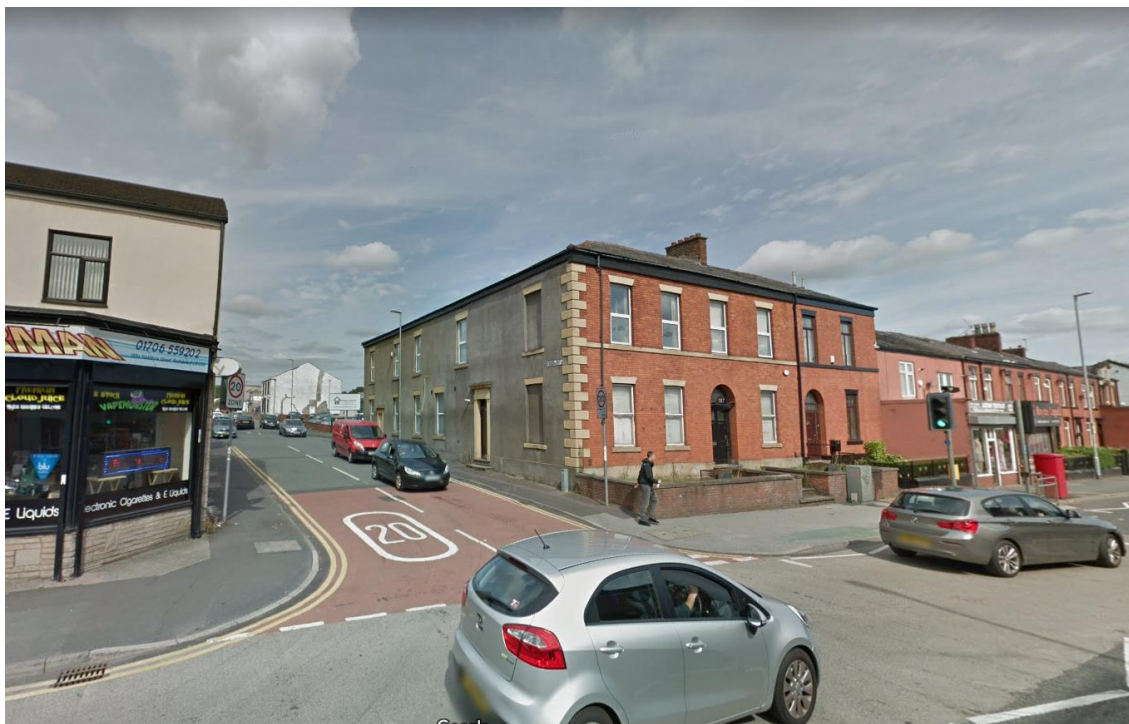
Photo above shows the front and side elevations of the application property.
