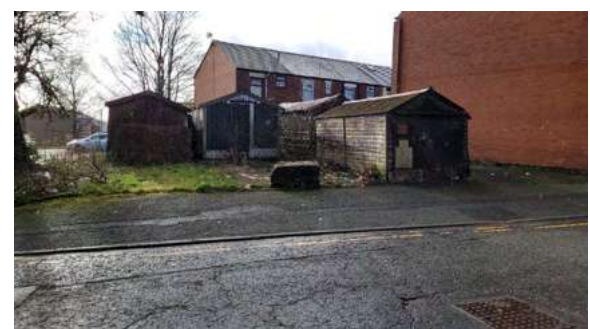
Block B – Existing Garages from the North
