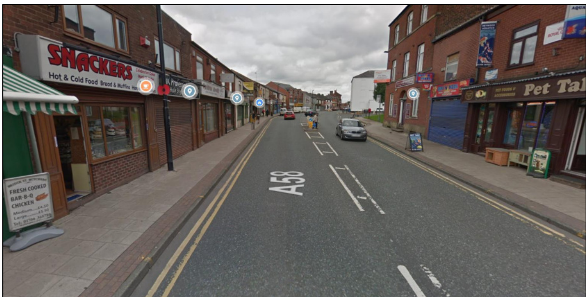
Figure 2.3: Local Highway Network - A58 Bridge Street
