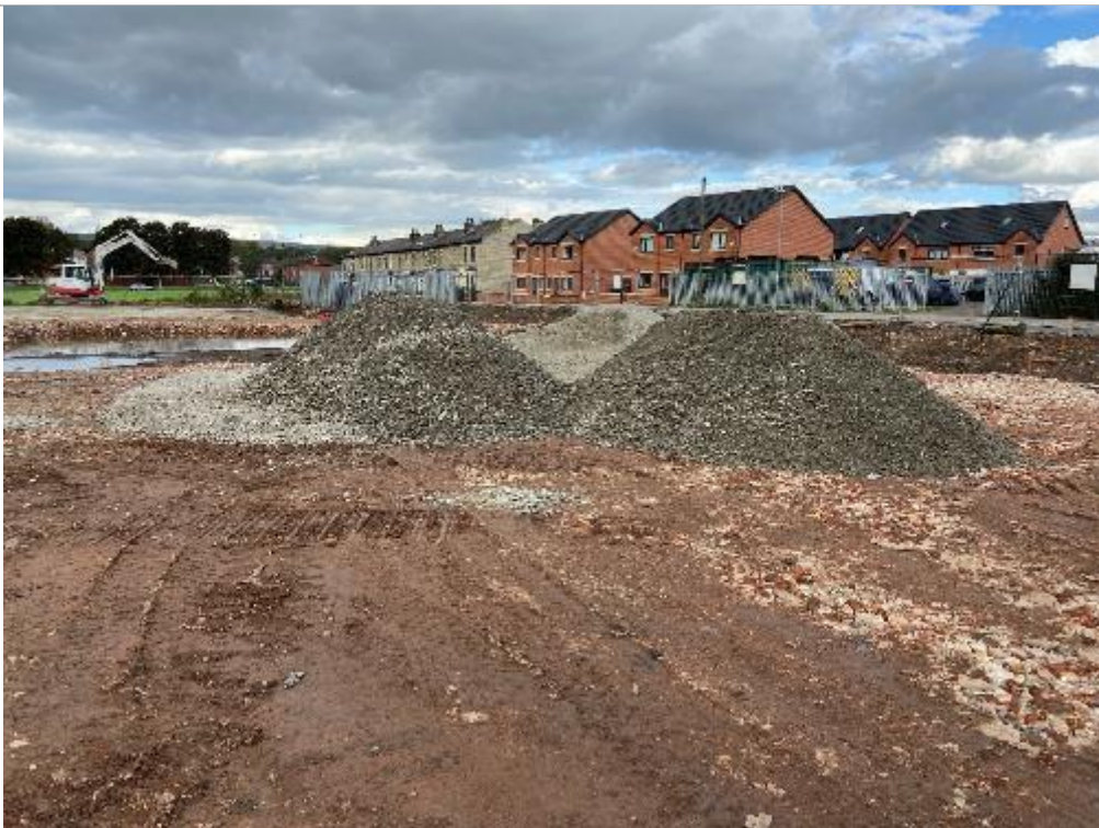
PLATE 32 IMPORTED MOT TYPE 1 STOCKPILE (FACING NORTH)
