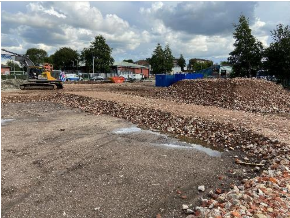
PLATE 28 6F2 ROAD BUILD UP IN CENTRE OF SITE (FACING SOUTH)
