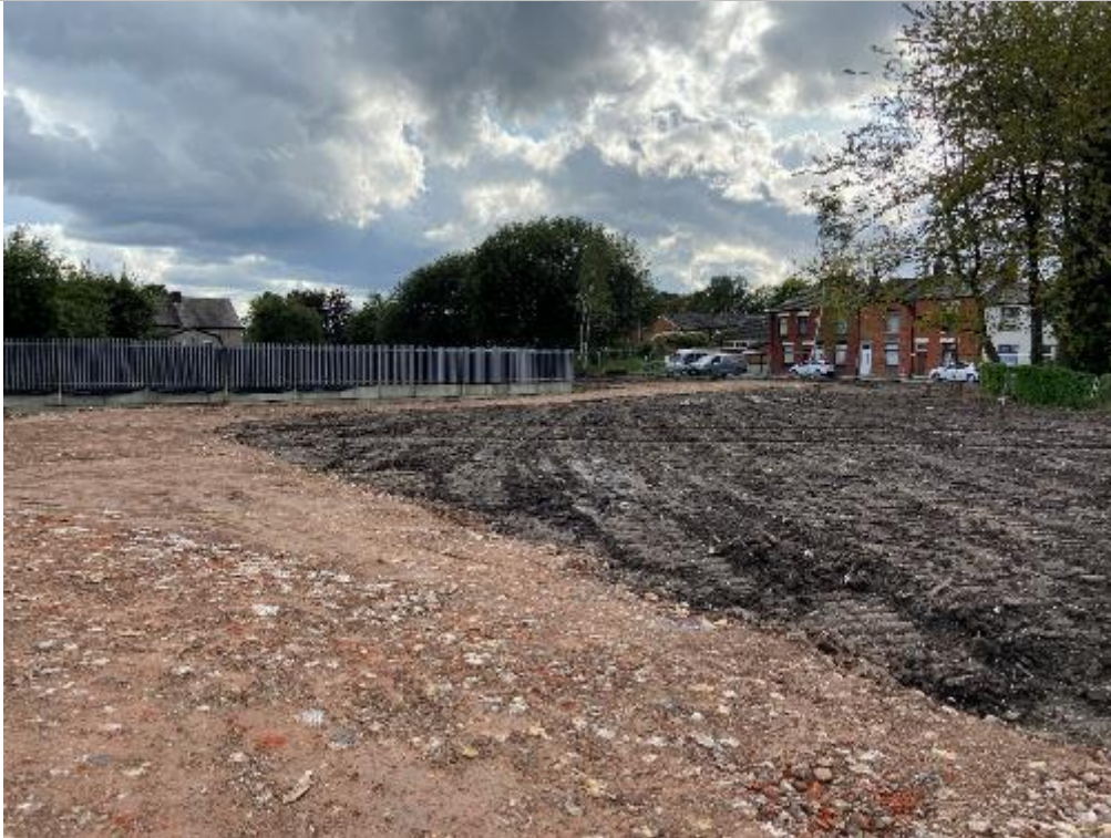
PLATE 29 6F2 ROAD BUILD UP IN SOUTH PART OF SITE (FACING SOUTHWEST)
