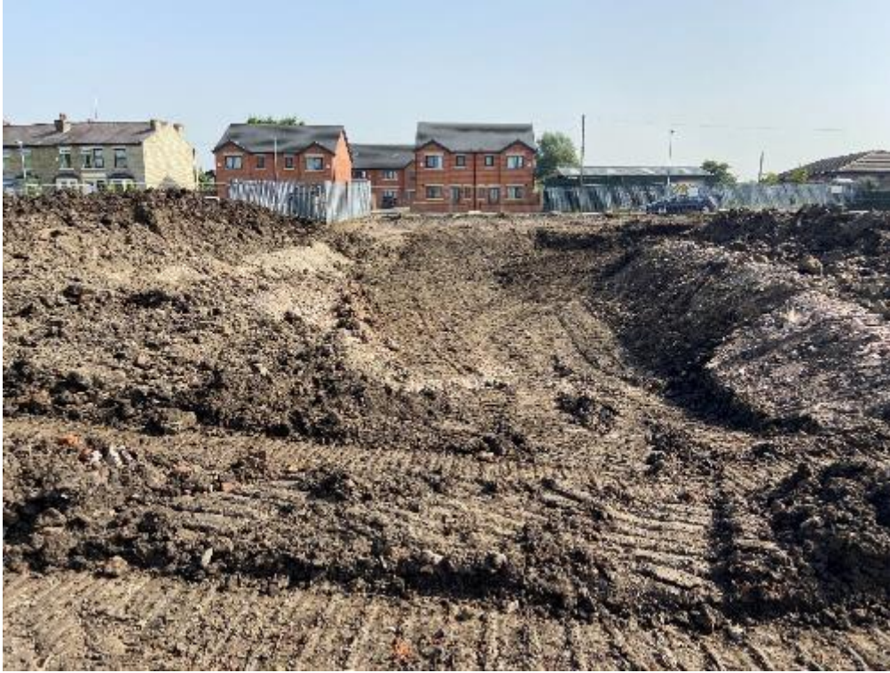
PLATE 21 SOFT SPOT EXCAVATION IN NORTH PART OF SITE, PENDING BACKFILL (FACING EAST)
