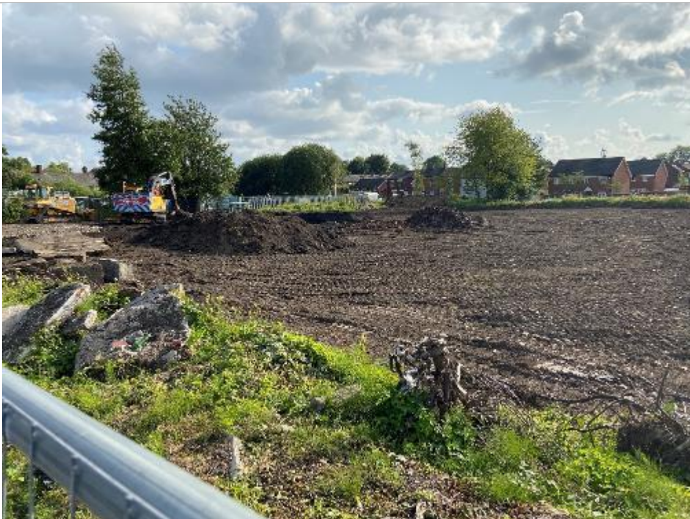
PLATE 4 VEGETATION STRIP ACROSS SITE (FACING SOUTHWEST)
