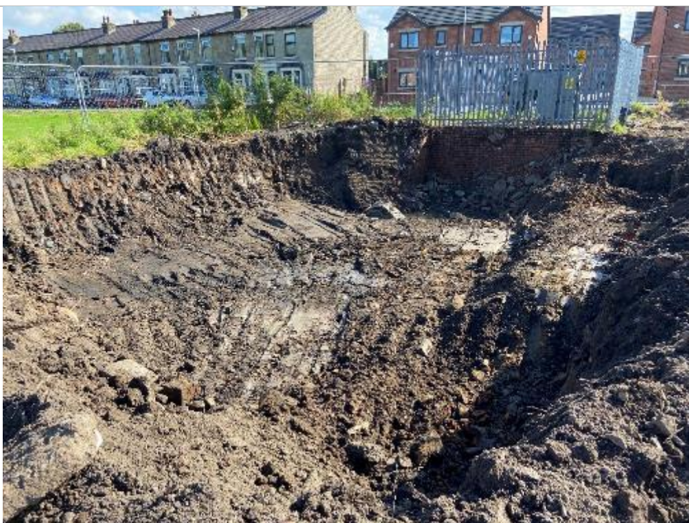
PLATE 14 TURNOVER / CUT/FILL WORKS IN NORTH PART OF SITE (FACING NORTHEAST)
