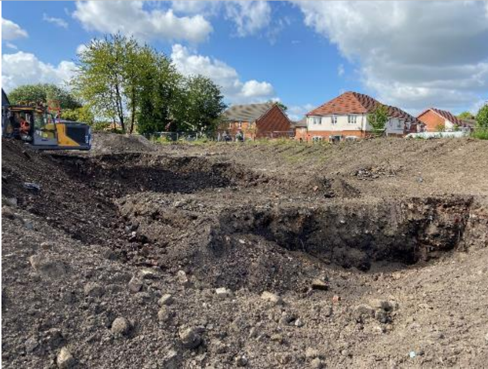
PLATE 10 EXCAVATION OF FRAGMENTISER WASTE IN NORTHWEST PART OF SITE (FACING SOUTH)
