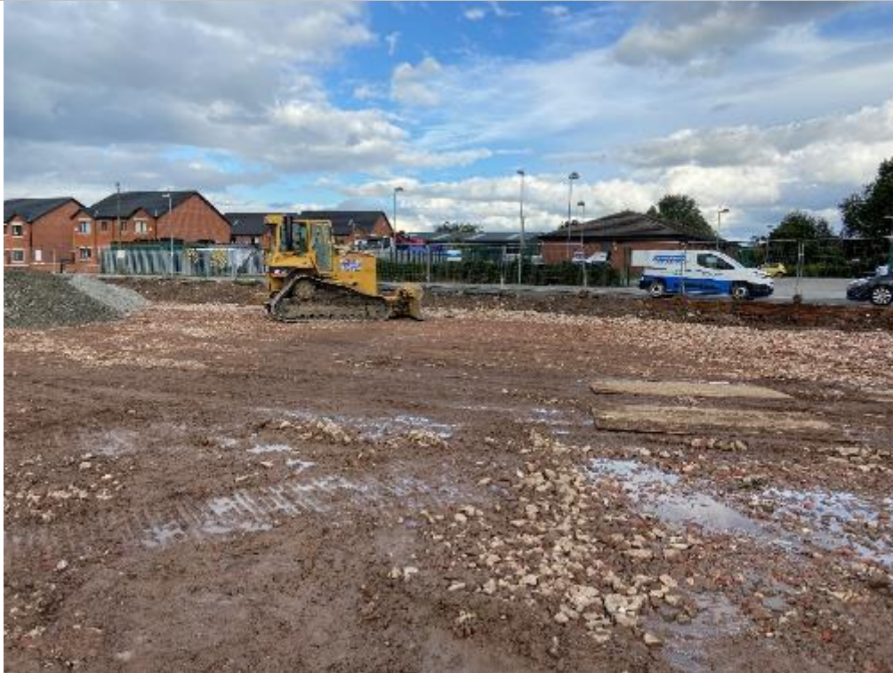
PLATE 25 SHOWROOM RAFT WITH 6F2 BUILD UP (FACING EAST)
