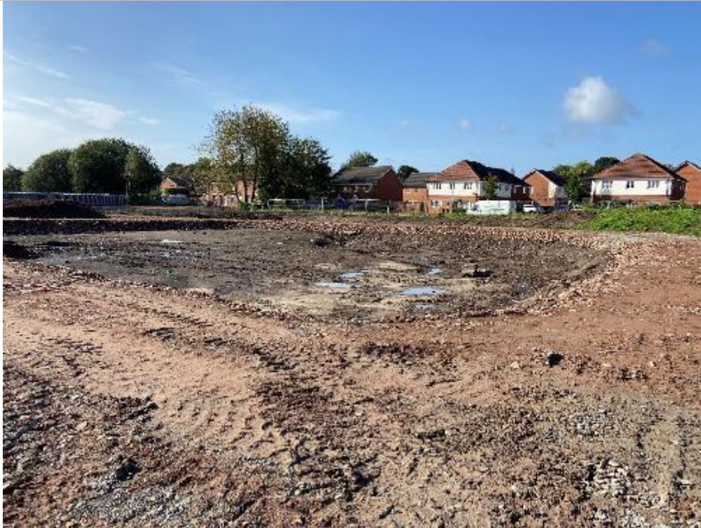
PLATE 27 6F2 ROAD BUILD UP IN NORTH PART OF SITE (FACING WEST)
