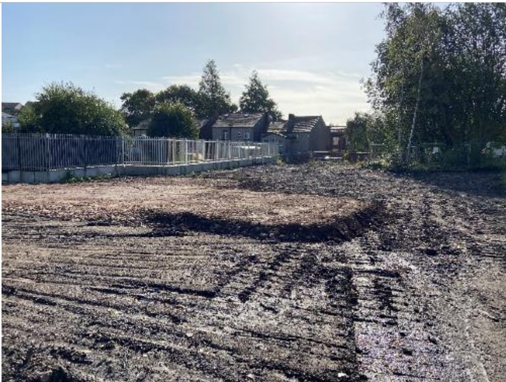
PLATE 30 6F2 ROAD BUILD UP IN SOUTHWEST PART OF SITE (FACING SOUTH)
