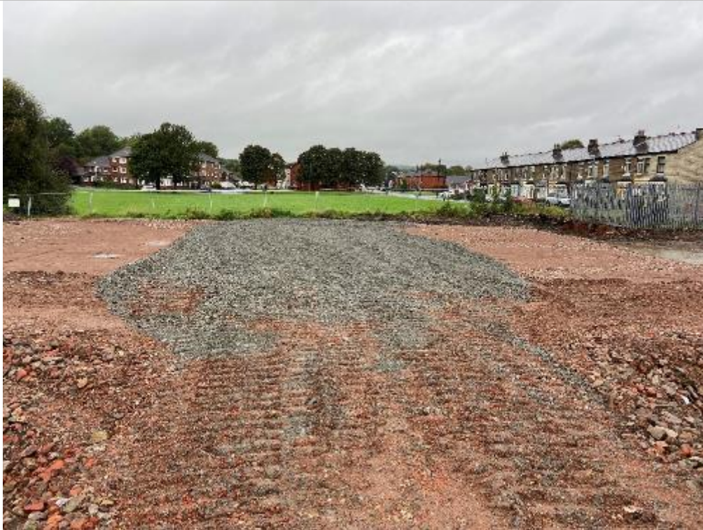
PLATE 23 WORKSHOP RAFT WITH 6F2 BUILD UP (FACING NORTH)
