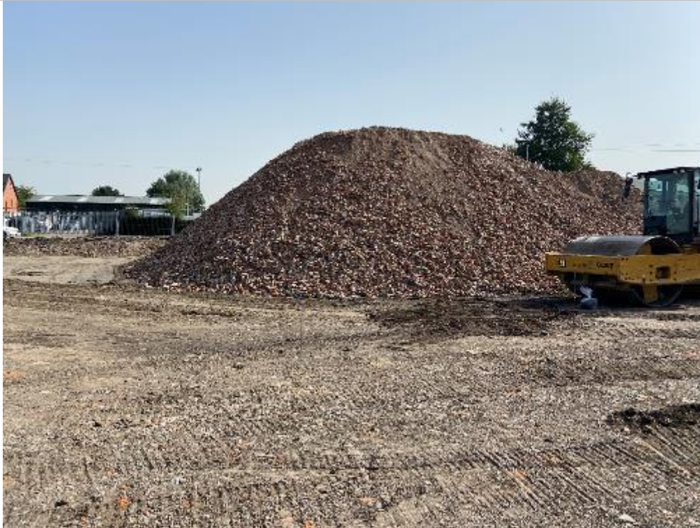
PLATE 19 6F2 STOCKPILE FOLLOWING CRUSHING (FACING EAST)
