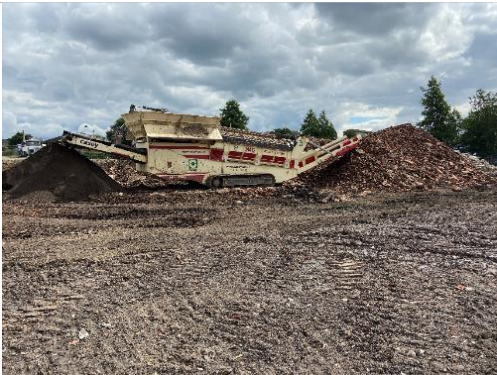
PLATE 16 PROCESSING MADE GROUND AND 6F2 STOCKPILE PENDING CRUSHING (FACING EAST)
