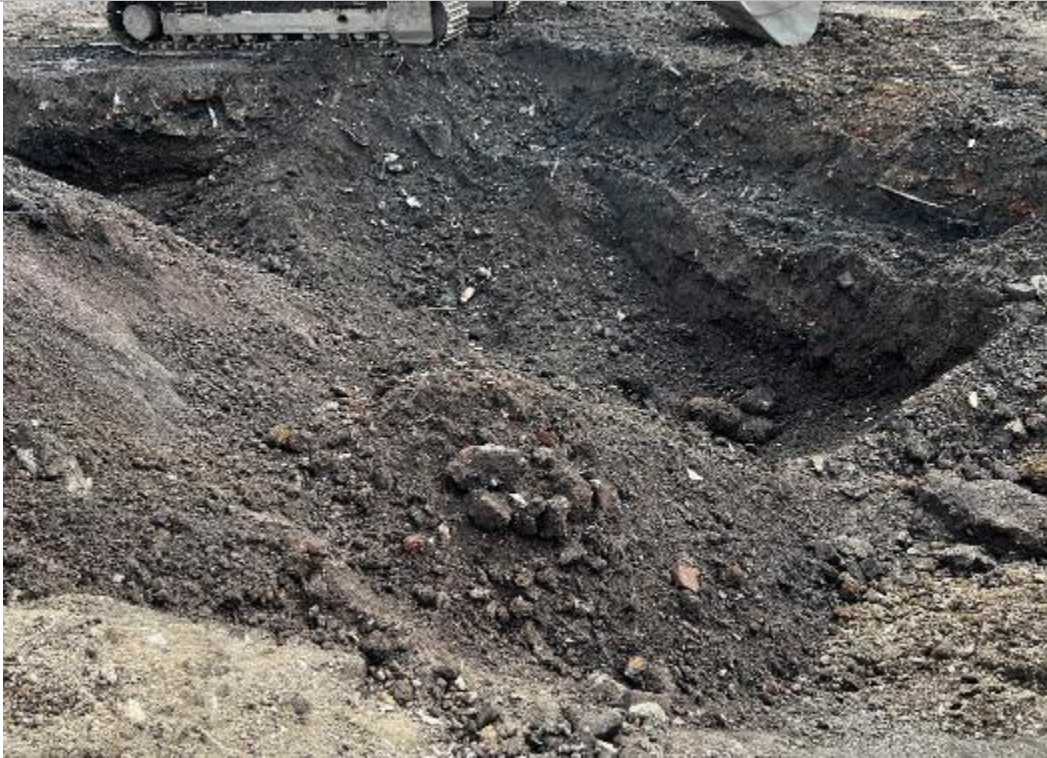
PLATE 8 EXCAVATION OF FRAGMENTISER WASTE IN NORTHWEST PART OF SITE (FACING SOUTH)
