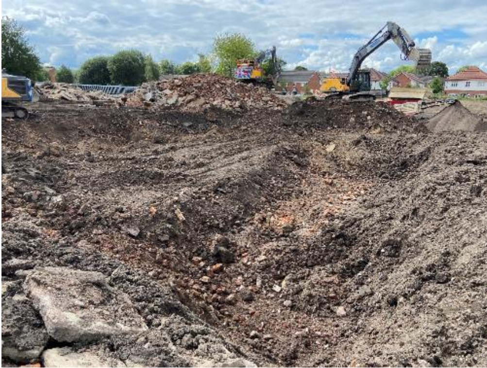
PLATE 17 TURNOVER / CUT/FILL WORKS IN CENTRAL PART OF SITE (FACING WEST)
