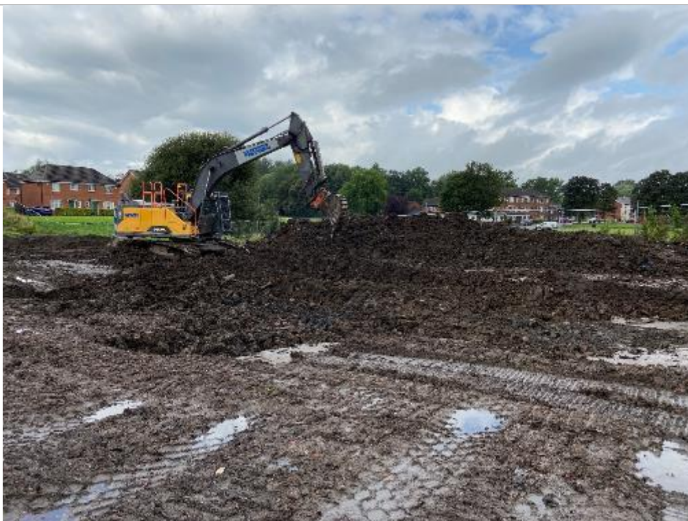
PLATE 20 EXCAVATION OF SOFT SPOT IN NORTH PART OF SITE (FACING NORTH)
