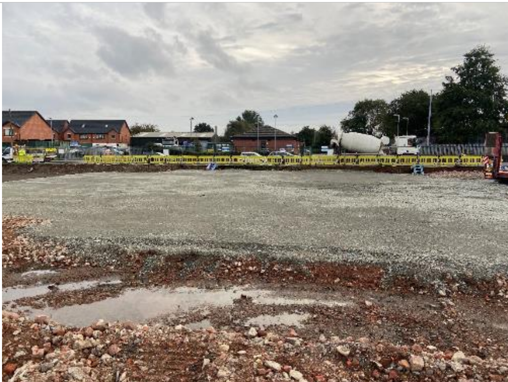
PLATE 26 SHOWROOM RAFT WITH MOT TYPE 1 BUILD UP (FACING EAST)
