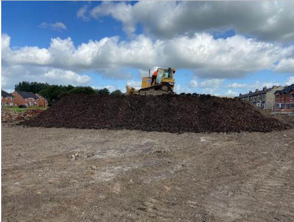
PLATE 15 PROCESSED MADE GROUND STOCKPILE (FACING NORTH)
