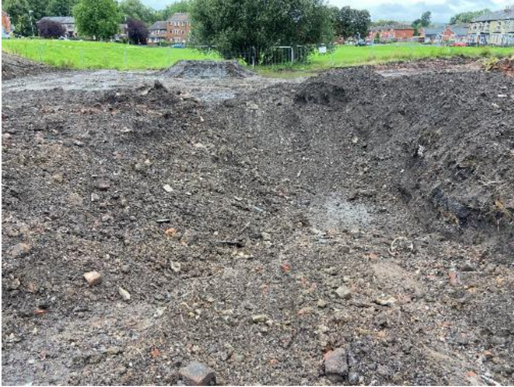
PLATE 7 EXCAVATION OF FRAGMENTISER WASTE IN NORTHWEST PART OF SITE (FACING NORTH)
