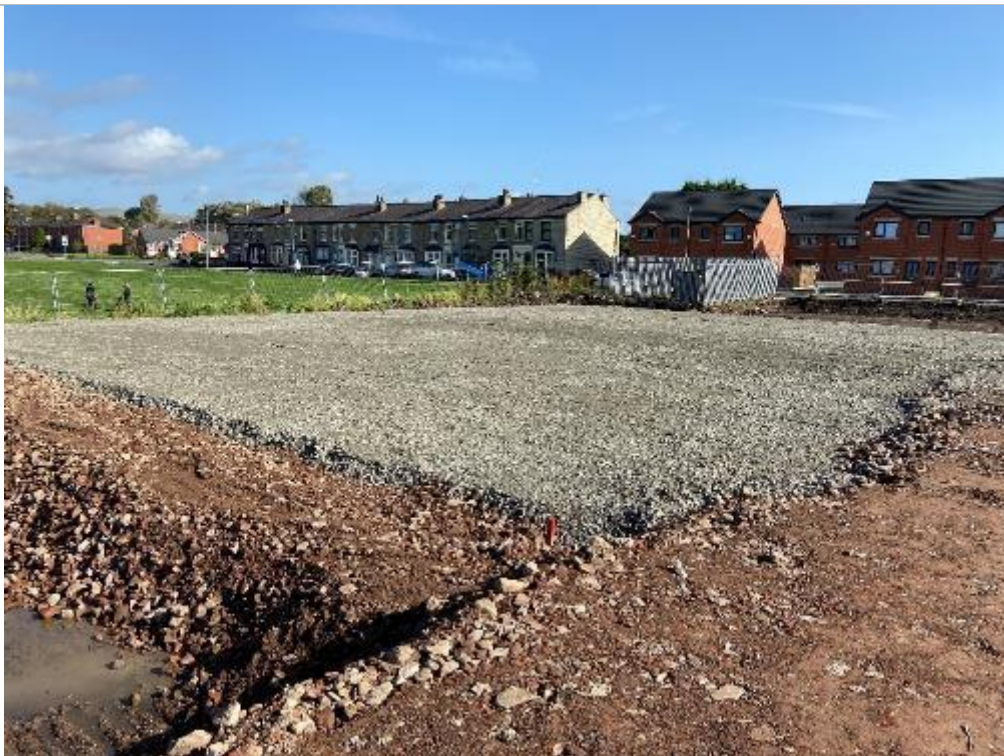
PLATE 24 WORKSHOP RAFT WITH MOT TYPE 1 BUILD UP (FACING NORTHEAST)
