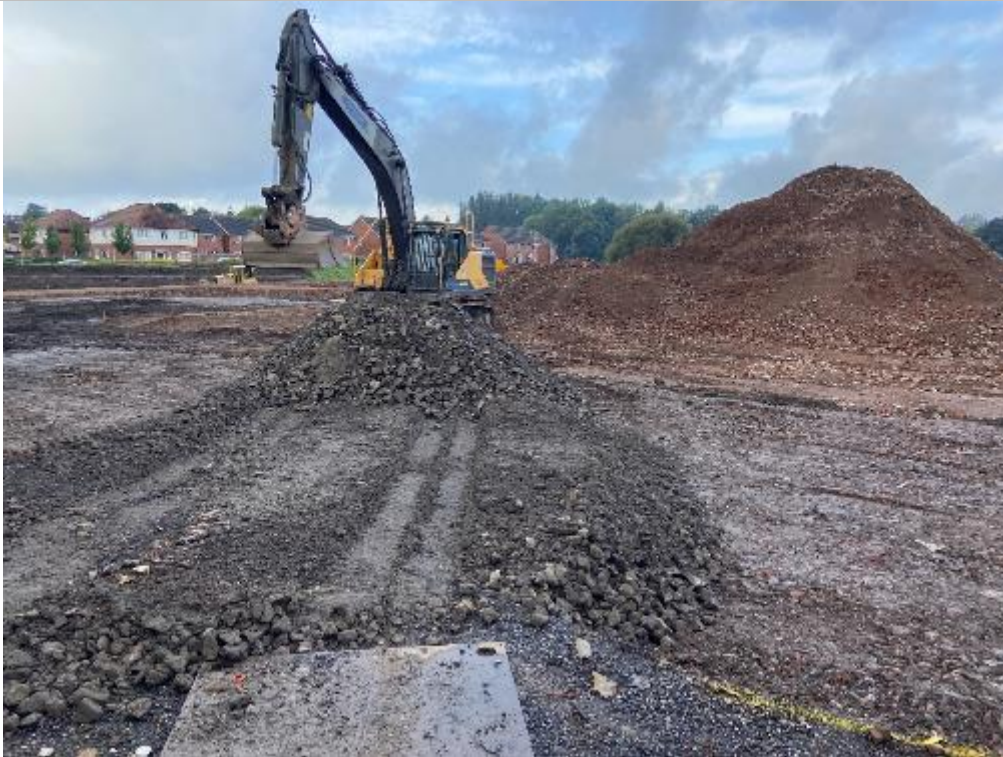
PLATE 31 IMPORTED 6F2 STOCKPILE (FACING NORTHWEST)
