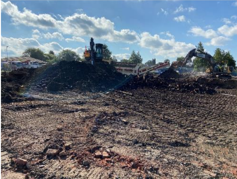
PLATE 13 PROCESSING AND STOCKPIILING OF MADE GROUND (FACING SOUTH)
