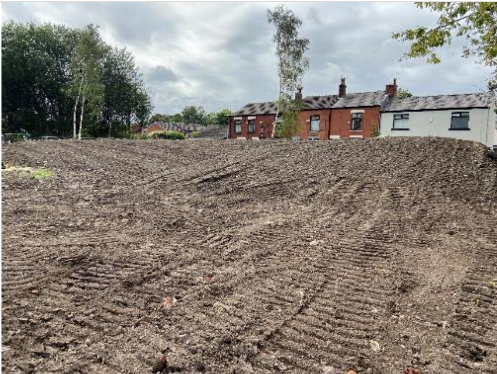
PLATE 6 TOPSOIL STOCKPILE IN SOUTHWEST CORNER (FACING SOUTHWEST)
