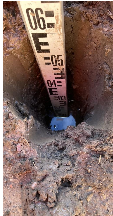
Plot 89: Internal View of excavation
