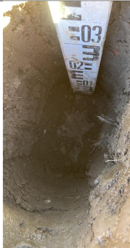
Plot 2: Internal View of excavation
