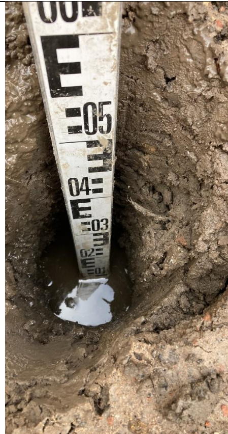
Plot 87: Internal View of excavation
