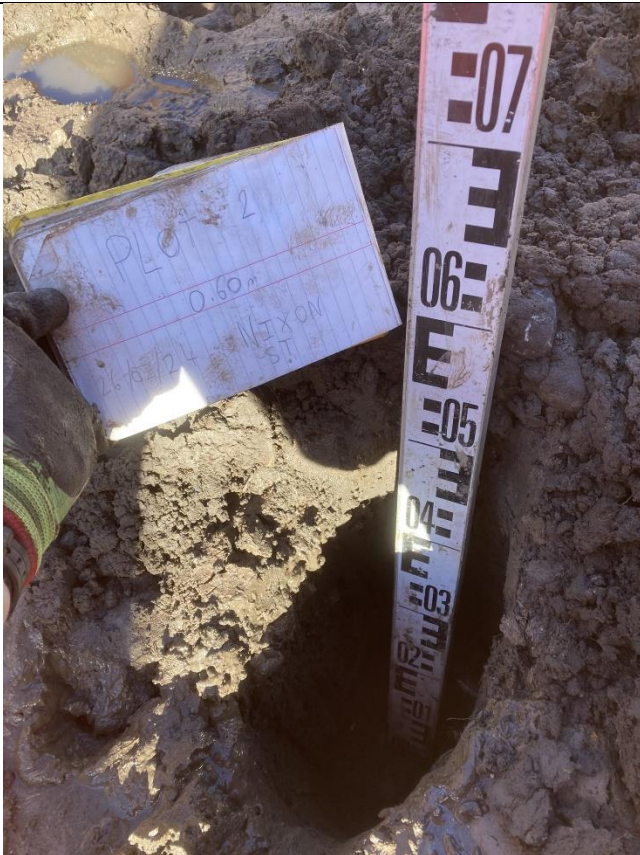
Plot 2: Overview of excavation
