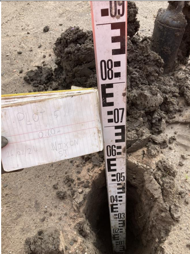
Plot 5: Overview of excavation
