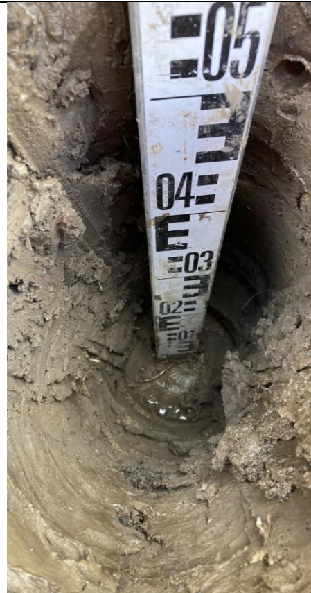
Plot 3: Internal View of excavation
