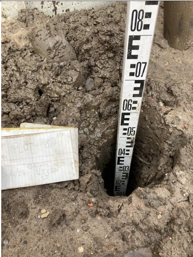
Plot 87: Overview of excavation
