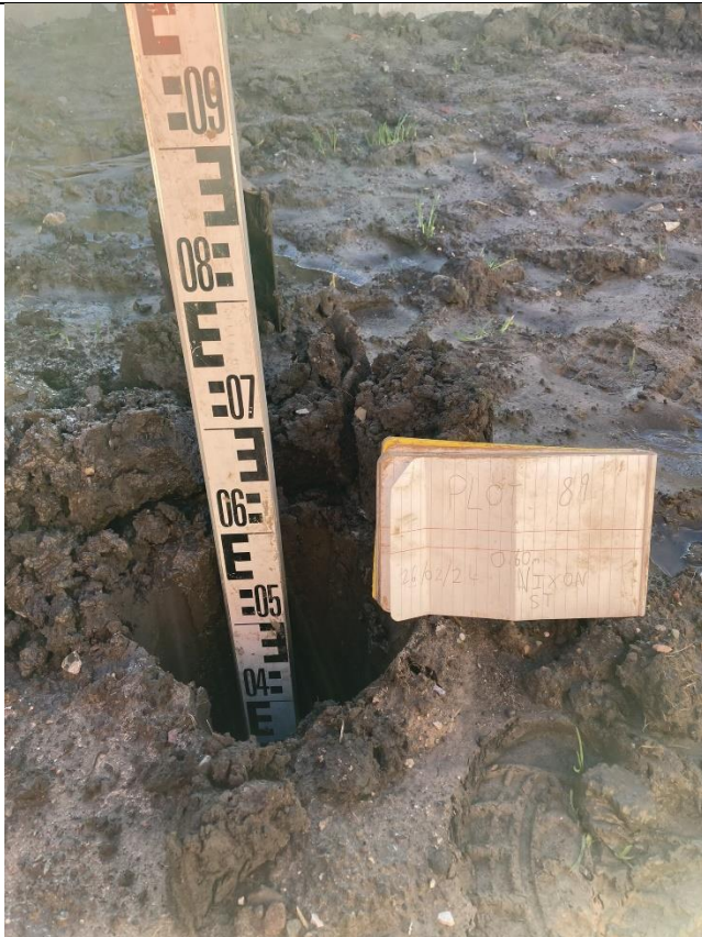
Plot 89: Overview of excavation
