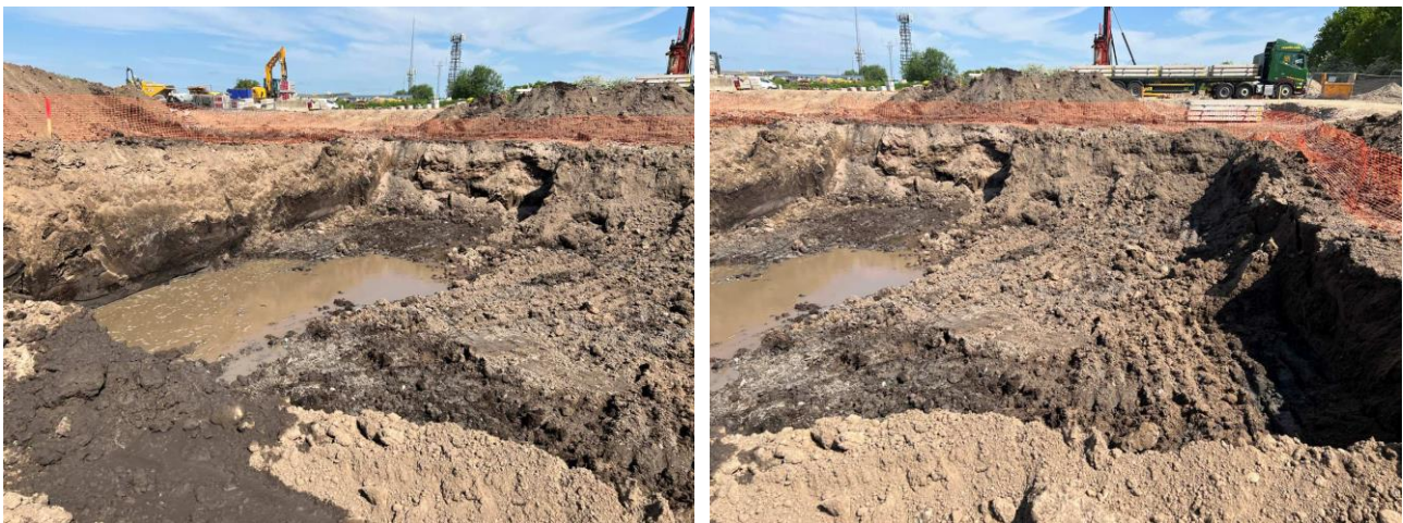
Photographs 203 and 204: Looking north west and northwards, verifying the excavation and removal of peat from the footprint of Plots 152 and garage, and the rear garden and garage of Plot 153. Note a thick layer of peat still present on the face of the excavation which at the time is noted to be the rear garden of Plot 154 and the eastern end of the garden of Plot 152, dated 24 th May 2023.
