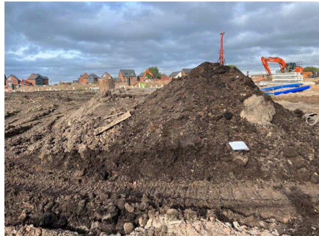
Photograph 100 (left) & 101 (right): Looking to the south, photograph 100 shows the road and sewer corridor construction in progress adjacent to Plots 136-142. Looking toward the west, photograph 101 shows peat that has been excavated from the adjacent road corridor and stockpiled on top of the proposed location of Plots 139-142, dated 19 th October 2022.
