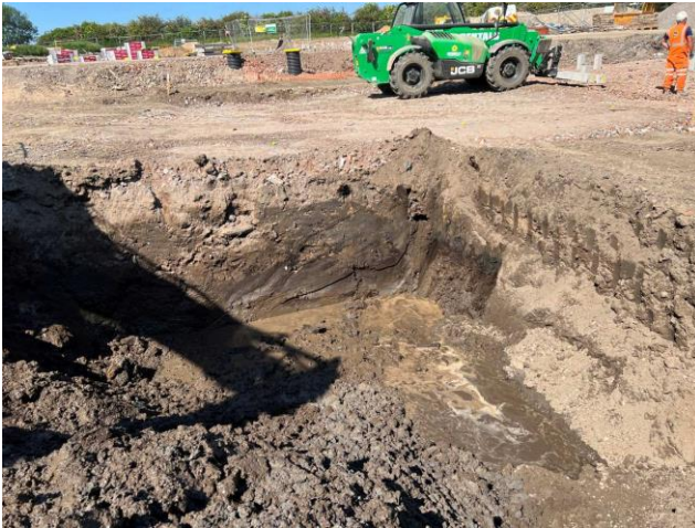
Photographs 220 and 221: Looking north-north eastwards showing progressive excavation of Plots 154 and 155's rear gardens and continued exposure of fibrous peat in the rear garden and rear wall of proposed Plot 154, dated 5 th June 2023.
