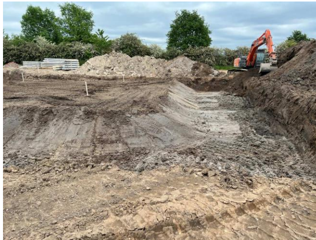
Photograph 217: Looking eastwards at the excavation spanning the remainder of Plot 150 and progressive backfill, dated 1 st June 2023.
