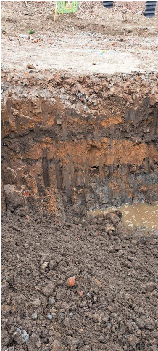
Photographs 222 and 223: Looking north-north eastwards showing the removal of the last remaining dark area of fibrous peat from the rear of Plot 154, dated 5 th June 2023.
