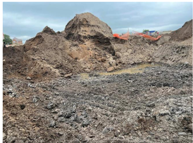
Photographs 215 and 216: Looking westwards at the progressive removal into the gardens of Plots 150 and 151. Remnant fibrous peat was still present beneath the loose spoil, dated 31 st May 2023.
