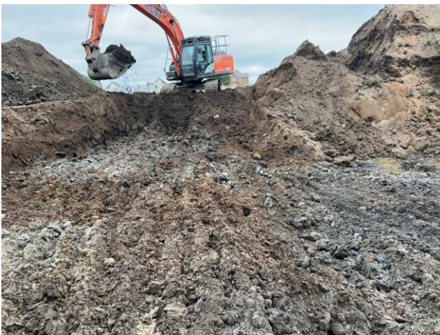
Photographs 215 and 216: Looking westwards at the progressive removal into the gardens of Plots 150 and 151. Remnant fibrous peat was still present beneath the loose spoil, dated 31 st May 2023.
