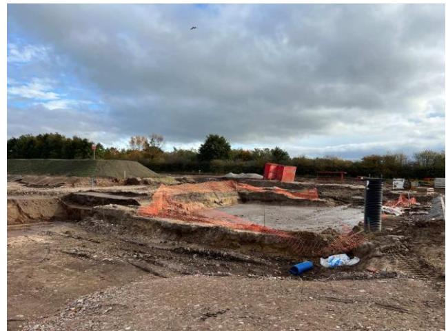
Photographs 201 and 202: Looking at a reduced level dig to accommodate pile mats for Plots 144-148 on 19 th October 2022, where peat was proven not to be present.
