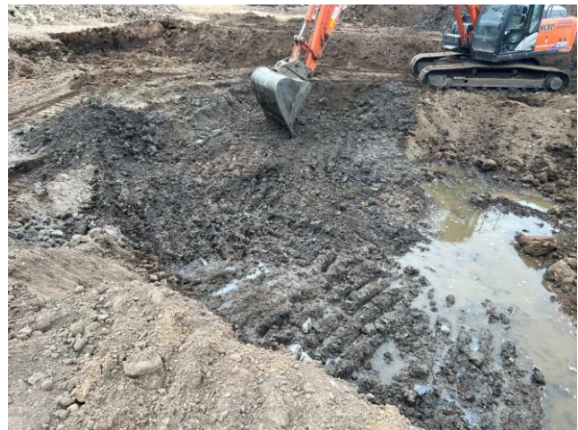
Photographs 213 and 214: Looking south east into the extent of excavation spanning Plot 151 and the right side of Plot 150. A band or pocket of re-worked peat between 200-300mm thick was present at 0.5m depth to the front of the right side of Plot 150 only, shown in the corner of the excavation in photograph 213, dated 31 st May 2023.
