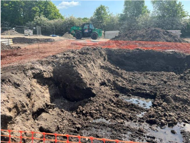
Photographs 205 and 206: Same excavation as photographs 203 and 204 looking westwards. The opposite face of the excavation is along the line of the proposed shared drive to the front of Plot 152. A layer of peat approximately 200-300mm thick was observed on the north face to the left, however the layer of peat appears to have disappeared to the east under the shared drive, dated 24 th May 2023.
