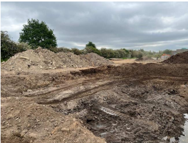
Photographs 213 and 214: Looking south east into the extent of excavation spanning Plot 151 and the right side of Plot 150. A band or pocket of re-worked peat between 200-300mm thick was present at 0.5m depth to the front of the right side of Plot 150 only, shown in the corner of the excavation in photograph 213, dated 31 st May 2023.
