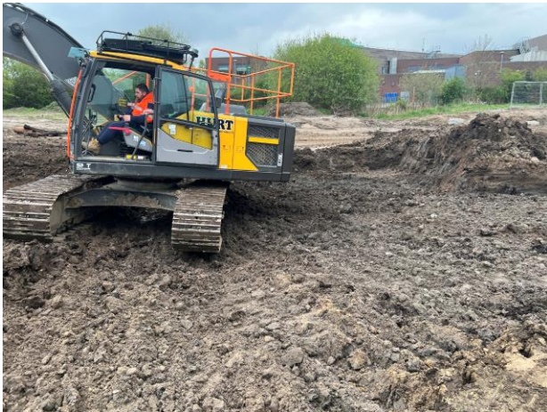
Photograph 108 (left) & 109 (right): Firstly, 108 shows the completed extent of the peat removal in the area of Plots 140-142 along the eastern face of the excavation. Looking in a northerly direction, photograph 109 shows the western most face of the excavation following the completed removal of remaining peat, dated 28 th April 2023.
