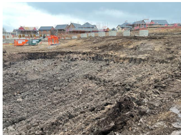
Photograph 106 (left) & 107 (right): Looking in a westerly direction, photograph 106 shows the completed extent of the peat removal in Plots 140-142, revealing the sands at the base. Looking in a south westerly direction, photograph 107 shows peat removal during excavation, with a thin band of peat progressively removed along the western face of the excavation, dated 28 th April 2023.
