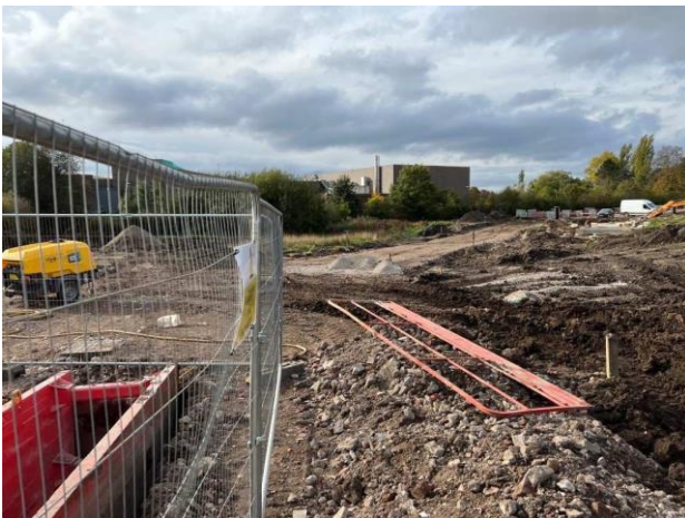
Photograph 100 (left) & 101 (right): Looking to the south, photograph 100 shows the road and sewer corridor construction in progress adjacent to Plots 136-142. Looking toward the west, photograph 101 shows peat that has been excavated from the adjacent road corridor and stockpiled on top of the proposed location of Plots 139-142, dated 19 th October 2022.
