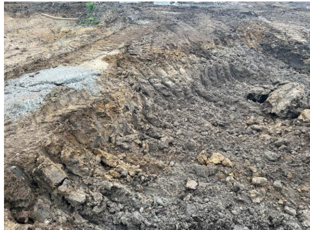
Photograph 108 (left) & 109 (right): Firstly, 108 shows the completed extent of the peat removal in the area of Plots 140-142 along the eastern face of the excavation. Looking in a northerly direction, photograph 109 shows the western most face of the excavation following the completed removal of remaining peat, dated 28 th April 2023.
