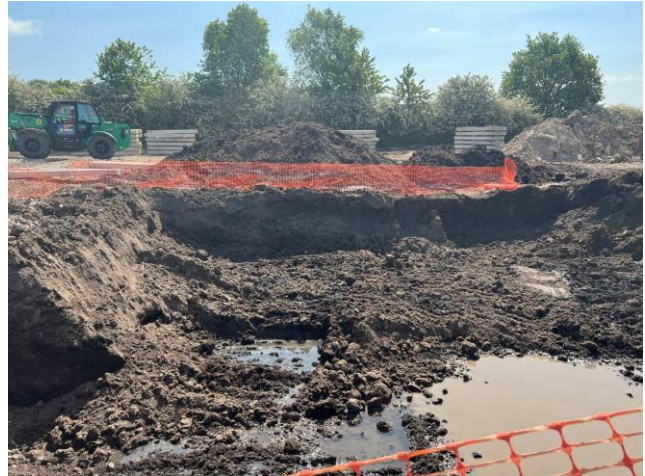
Photographs 205 and 206: Same excavation as photographs 203 and 204 looking westwards. The opposite face of the excavation is along the line of the proposed shared drive to the front of Plot 152. A layer of peat approximately 200-300mm thick was observed on the north face to the left, however the layer of peat appears to have disappeared to the east under the shared drive, dated 24 th May 2023.
