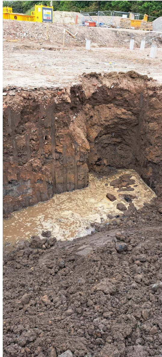
Photographs 222 and 223: Looking north-north eastwards showing the removal of the last remaining dark area of fibrous peat from the rear of Plot 154, dated 5 th June 2023.
