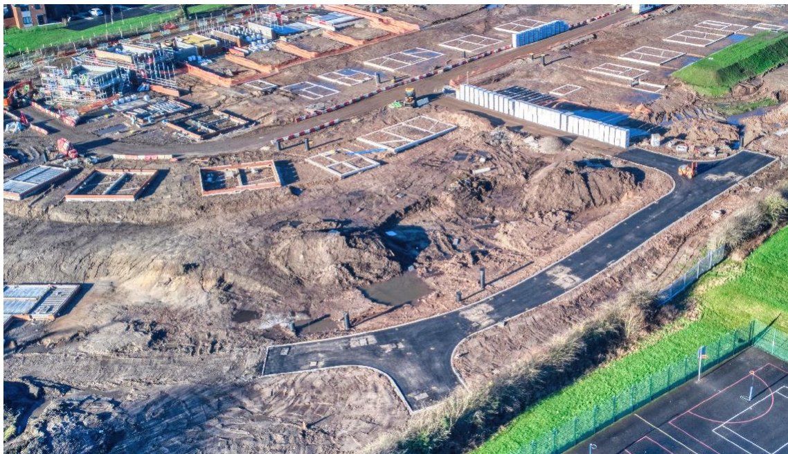
Photograph 104: Drone photograph showing progress of excavation and removal of peat by PAS, received by Coopers on 26 th January 2023.
