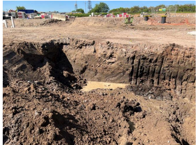
Photographs 220 and 221: Looking north-north eastwards showing progressive excavation of Plots 154 and 155's rear gardens and continued exposure of fibrous peat in the rear garden and rear wall of proposed Plot 154, dated 5 th June 2023.
