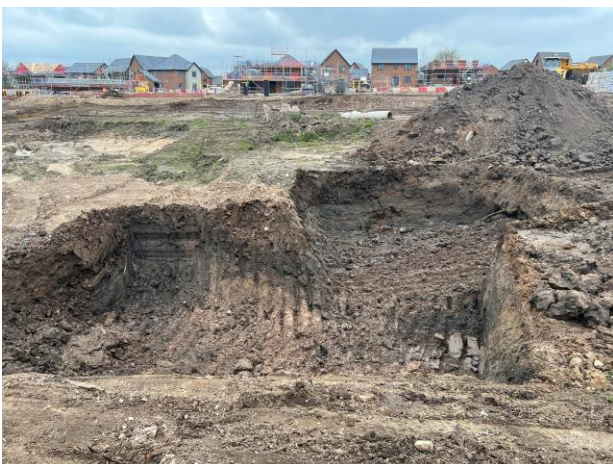
Photograph 106 (left) & 107 (right): Looking in a westerly direction, photograph 106 shows the completed extent of the peat removal in Plots 140-142, revealing the sands at the base. Looking in a south westerly direction, photograph 107 shows peat removal during excavation, with a thin band of peat progressively removed along the western face of the excavation, dated 28 th April 2023.
