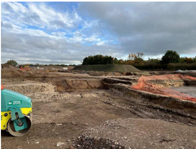
Photographs 201 and 202: Looking at a reduced level dig to accommodate pile mats for Plots 144-148 on 19 th October 2022, where peat was proven not to be present.
