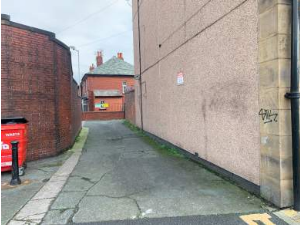
Plate 7 – Alleyway to the north of the 3-storey building, leading to courtyard area, looking west.
